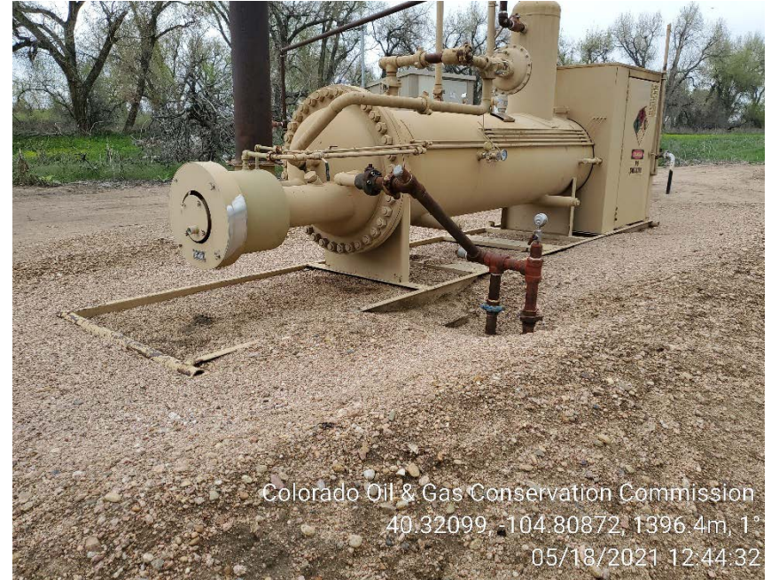
Edkam 5-34 separator anchoring
