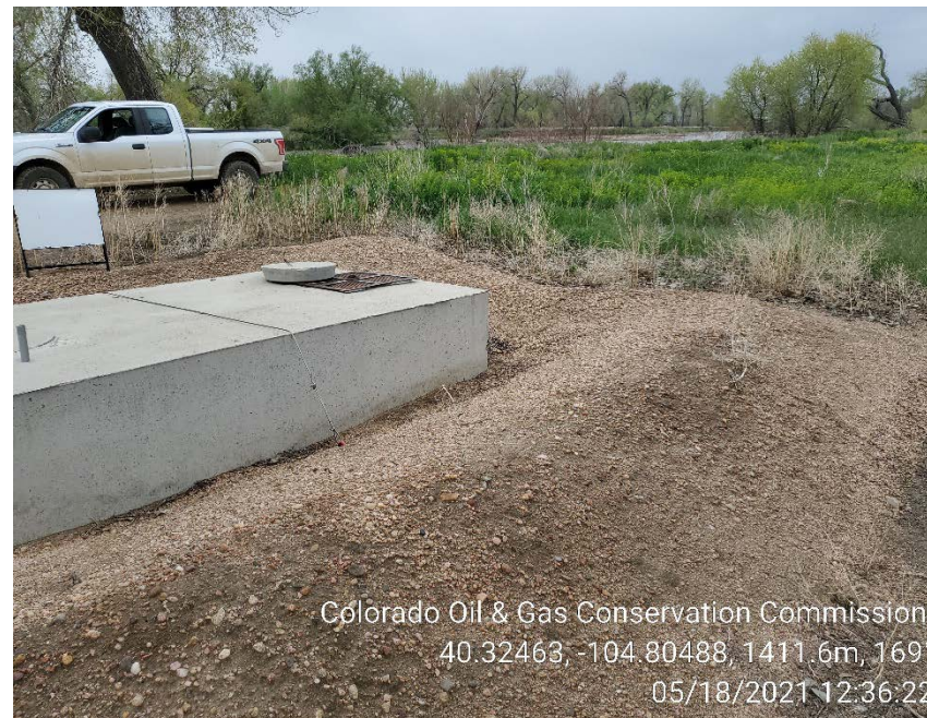
Produced water vault berm at Edkam 4-33
