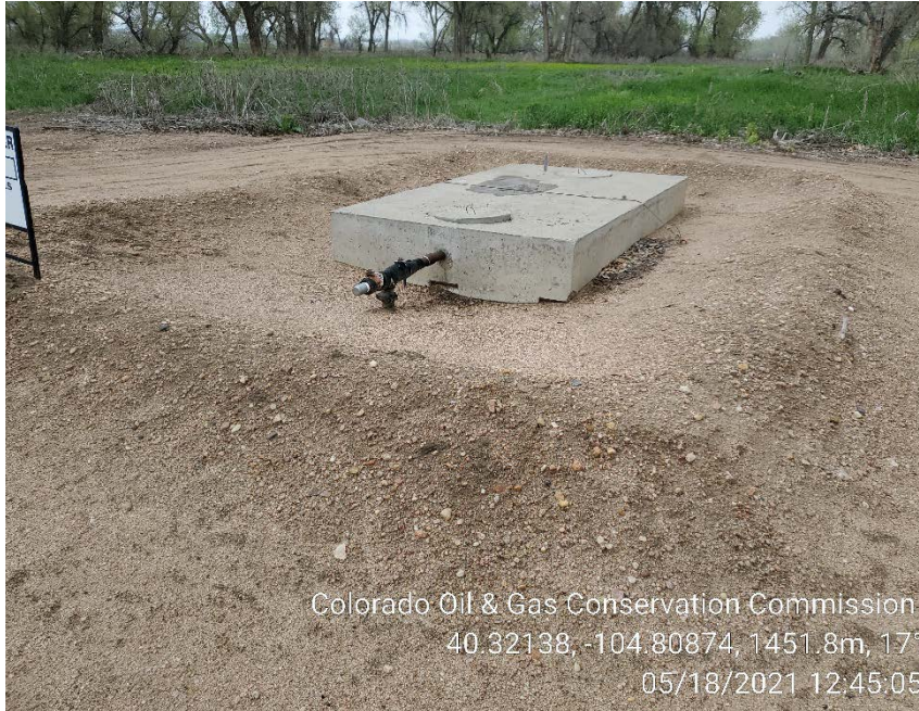
Produced water vault berm at Edkam 5-34
