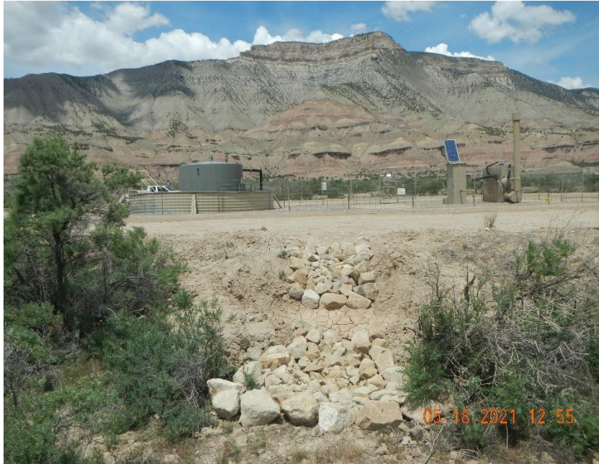
Check dam installed
