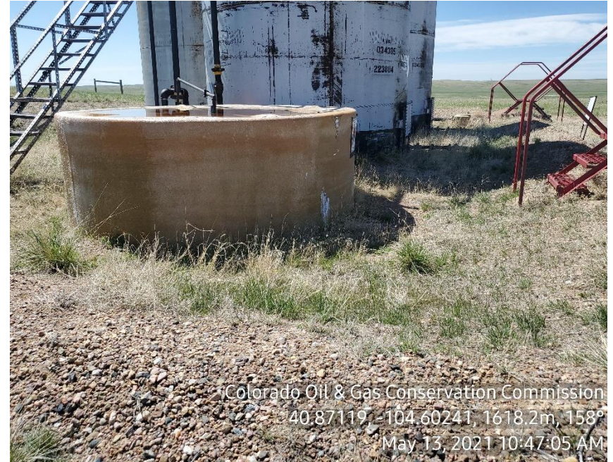
Photo 4: Weeds inside tank battery berm
