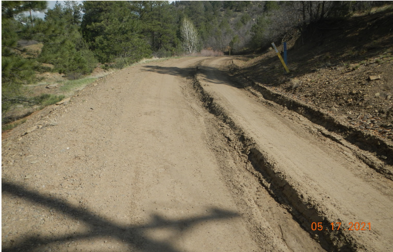
Photo 1. There is vehicle rutting along the main road. Areas of rutting need to be stabilized.
