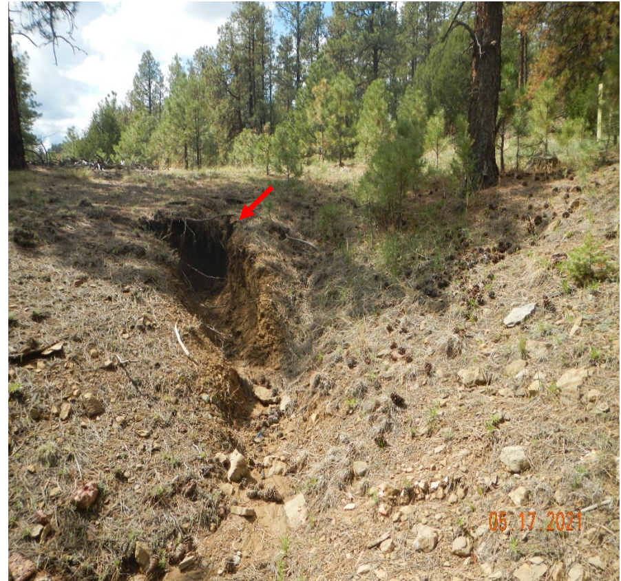
Photo 7. Stormwater directed from the road has caused a washout at area shown at red arrows. Lat/Long:37.09432,-104.94607
