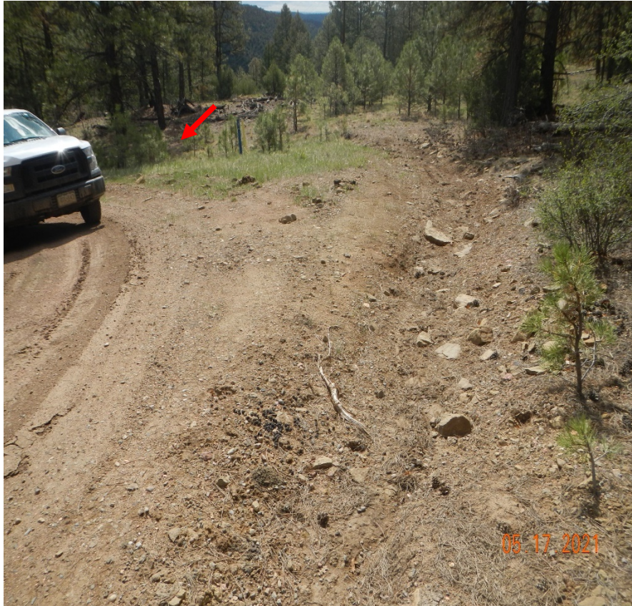
Photo 7. Stormwater directed from the road has caused a washout at area shown at red arrows. Lat/Long:37.09432,-104.94607
