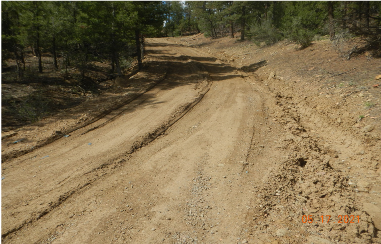
Photo 6. The vehicle rutting has not been repaired since previous inspection. Areas of the road are not stabilized and susceptible to further erosion.
