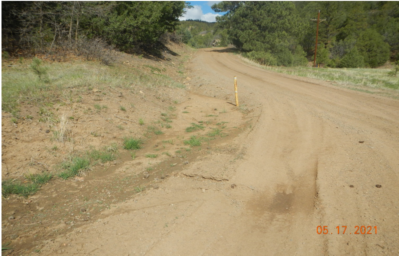
Photo 3. The culvert is filled in with sediment causing stormwater to flow down the road. All culverts need to be maintained. Previous corrective action was not performed.
