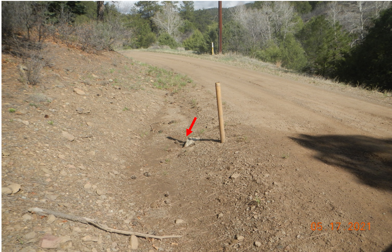
Photo 2. There is a plugged culvert along the main road (red arrow). Previous corrective action was not performed.
