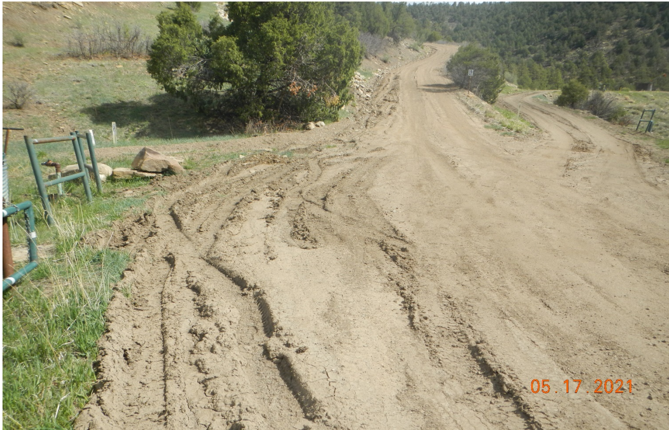
Photo 4. There is vehicle rutting off the side of the road., This area needs to be stabilized. BMP's are also needed along the steep grade of the road to prevent erosion.
