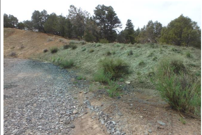
Northern Cut-Slope after Seeding
