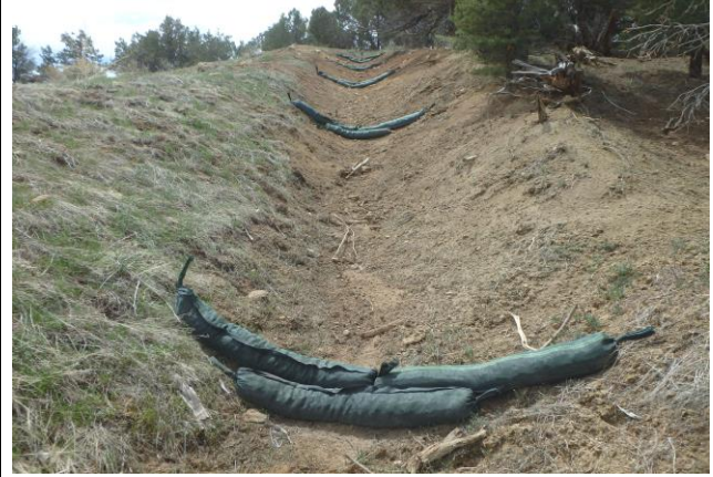
Rock Socks Installed in Northern Containment
