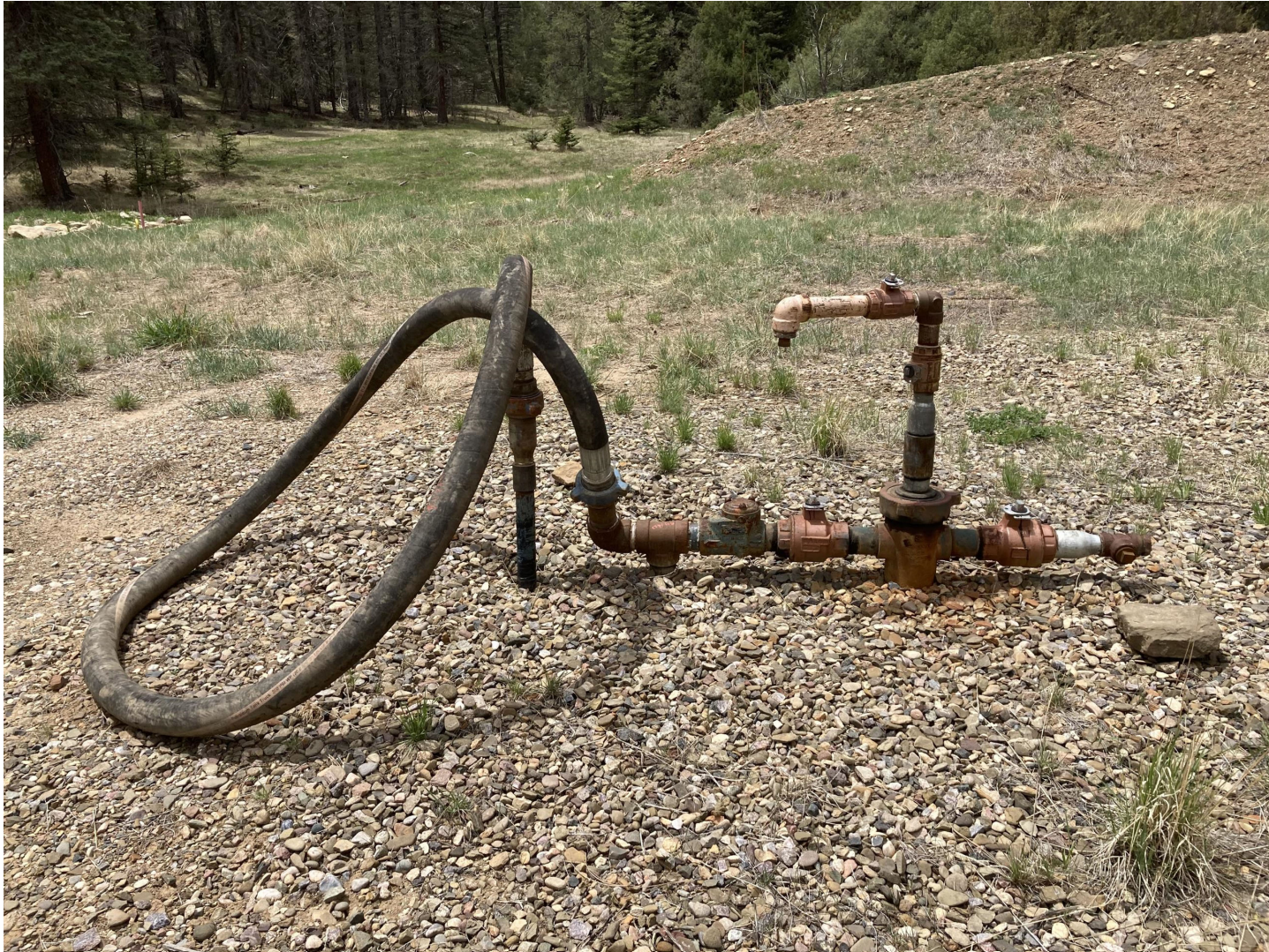
PHOTO 11: THE RISER IS A LOW PRESURE BY-PASS THAT ARE IN USE. THE RISER WAS LABELED AS TO IT'S FUNCTION.
