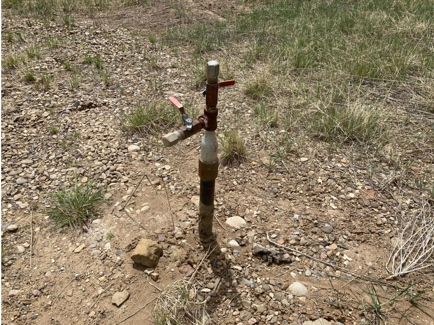
PHOTO 13: THE RISER IS FUEL LINE. THE RISER WAS LABELED AS TO IT'S FUNCTION.
