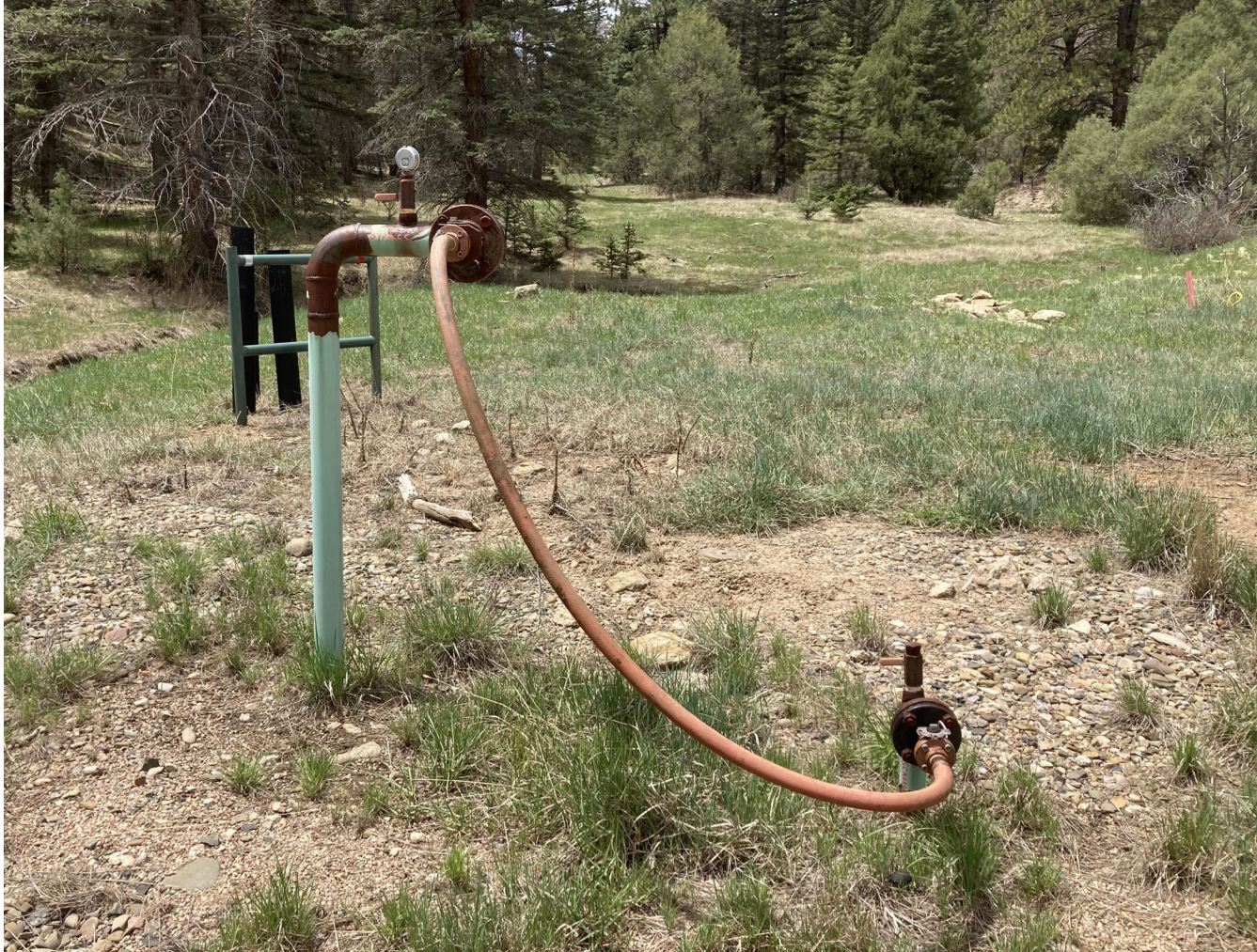
PHOTO 2: THE RISER'S ARE LOW PRESURE BY-PASS THAT ARE IN USE. EACH RISER WAS LABELED AS TO IT'S FUNCTION.
