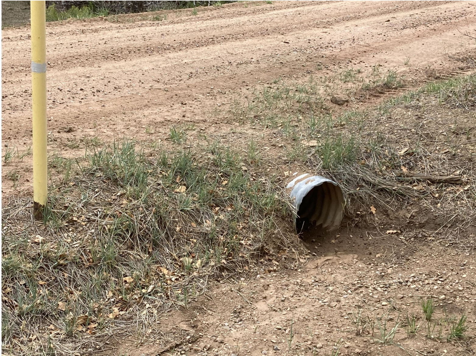
PHOTO 4: THE SEDIMENT ACCUMULATION WAS REMOVED FROM THE CULVERT INLET.
