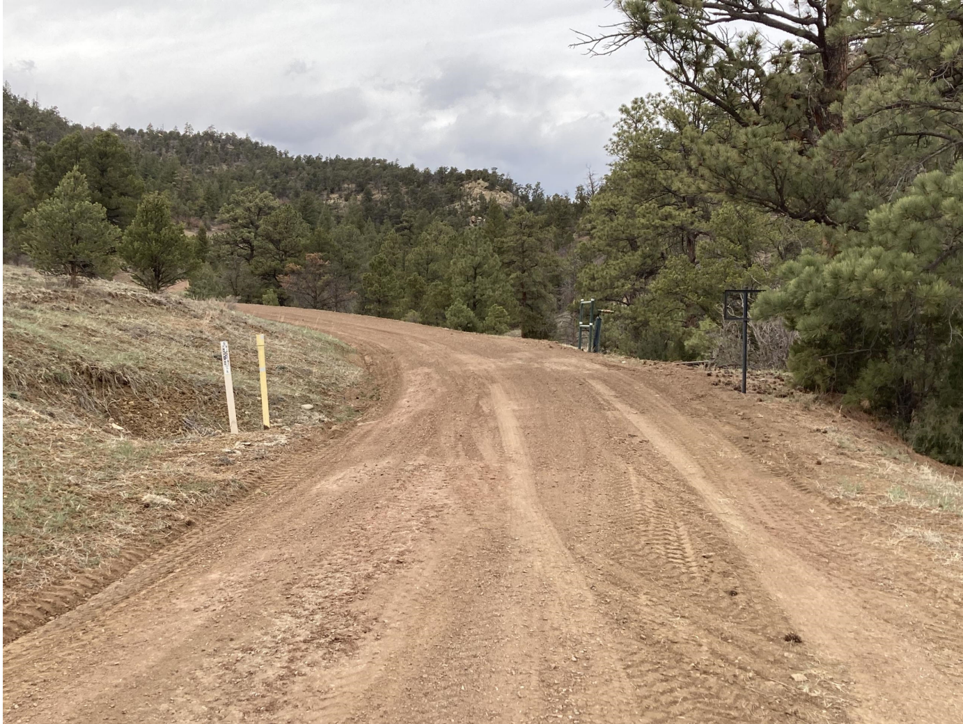
PHOTO 1: THE LEASE ROAD SURFACE IN LOPEZ CANYON WAS CROWNED TO CREATE SHEET FLOW AND ELIMINATE THE TIRE RUTS.
