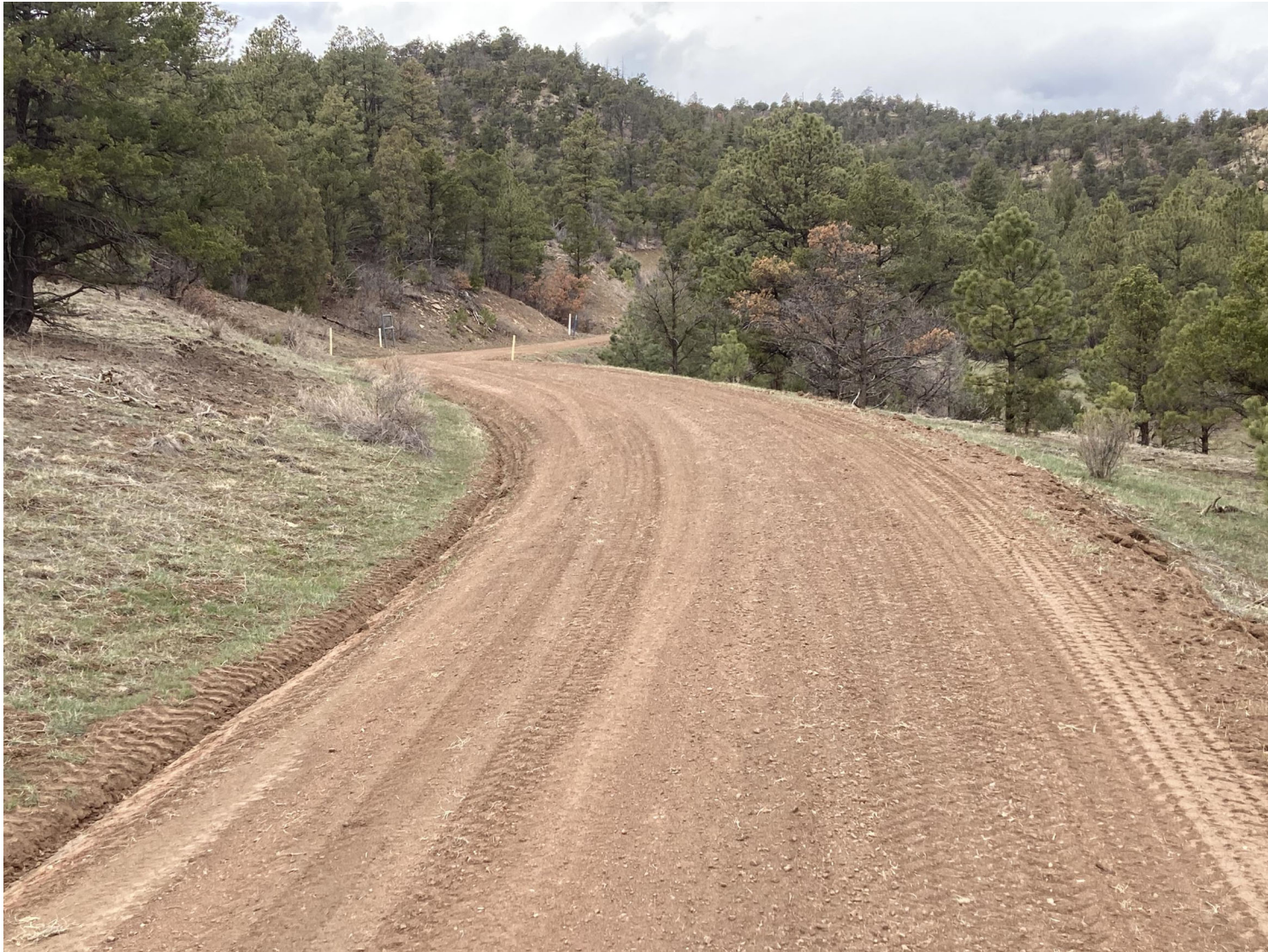
PHOTO 3: THE LEASE ROAD SURFACE IN LOPEZ CANYON WAS CROWNED TO CREATE SHEET FLOW AND ELIMINATE THE TIRE RUTS. THE BAR DITCH WAS DOMINATED TO RECEIVE STORMWATER RUN OFF FROM THE LEASE ROAD AND DIRECT RUN OFF TO THE CULVERT INLETS.
