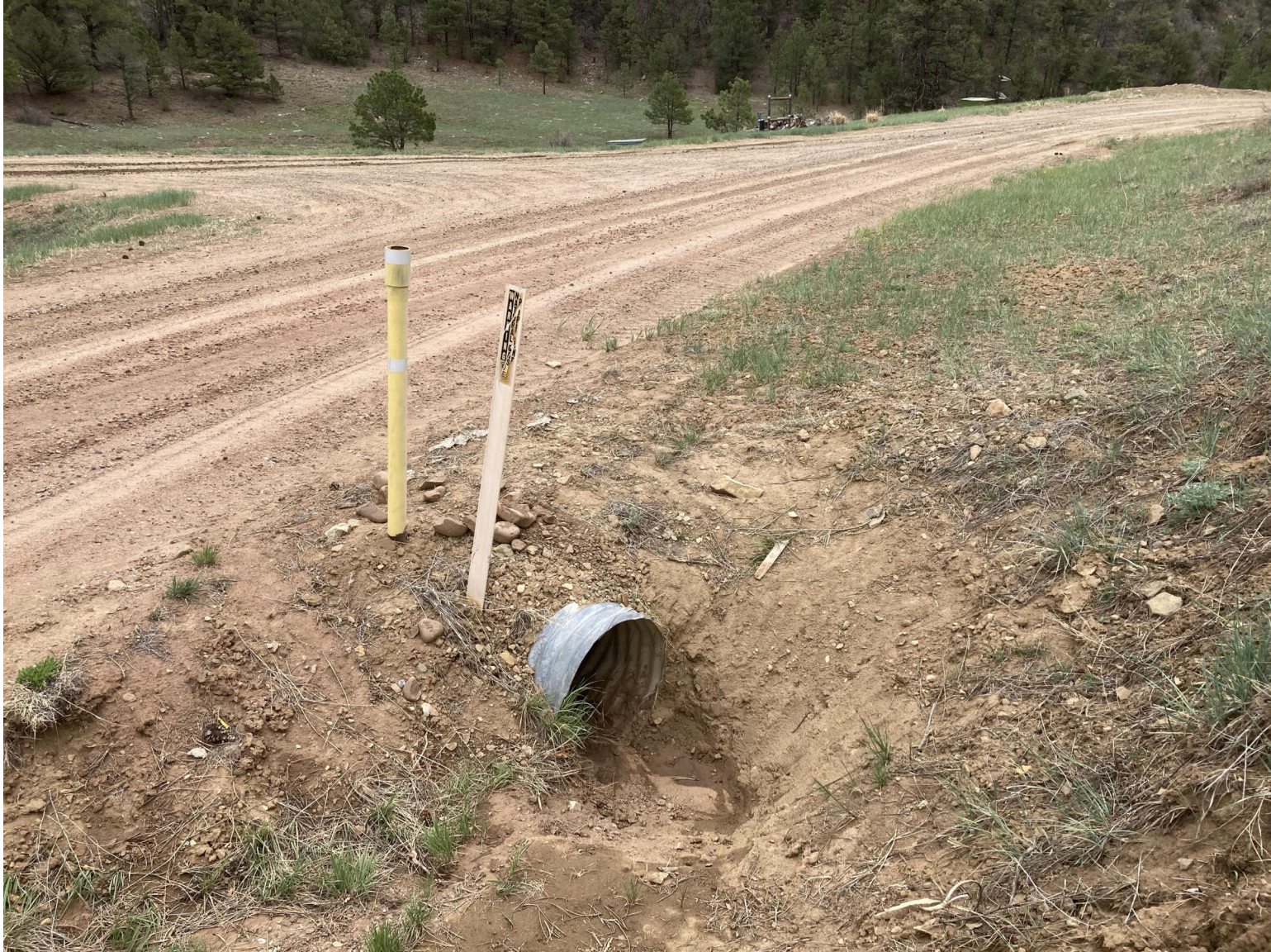
PHOTO 2: THE SEDIMENT ACCUMULATION WAS REMOVED FROM THE CULVERT INLET.
