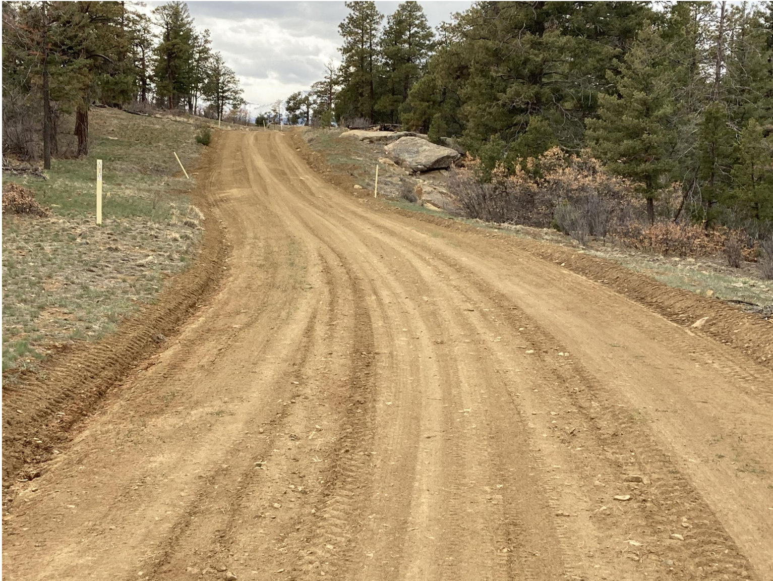
PHOTO 8: THE LEASE ROAD SURFACE IN LOPEZ CANYON WAS CROWNED TO CREATE SHEET FLOW AND ELIMINATE THE SURFACE EROSION.
