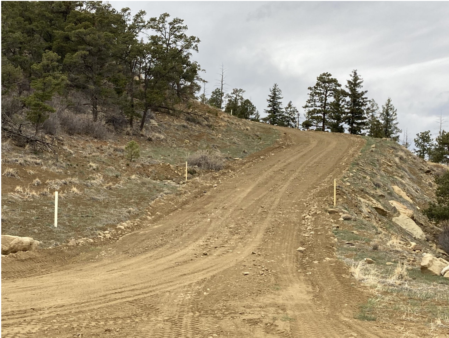
PHOTO 7: THE LEASE ROAD SURFACE IN LOPEZ CANYON WAS CROWNED TO CREATE SHEET FLOW AND ELIMINATE THE SURFACE EROSION.
