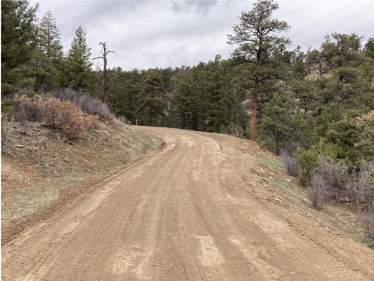
PHOTO 5: THE LEASE ROAD SURFACE IN LOPEZ CANYON WAS CROWNED TO CREATE SHEET FLOW AND ELIMINATE THE TIRE RUTS. THE BAR DITCH WAS DOMINATED TO RECEIVE STORMWATER RUN OFF FROM THE LEASE ROAD AND DIRECT RUN OFF TO THE CULVERT INLETS.
