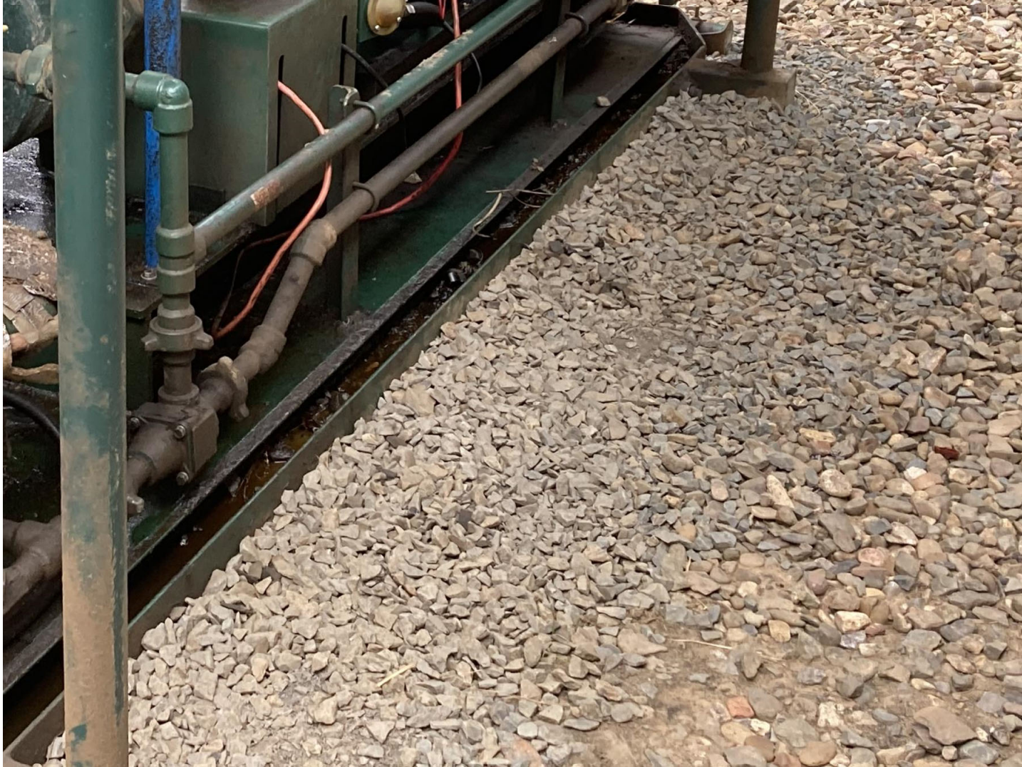
PHOTO 1: ALL FITTINGS ARE SECURLY FASTENED ON THE LIQUID RING COMPRESSOR. THE FLUID ACCUMULATION WAS REMOVED FROM THE CONTAINMENT.
