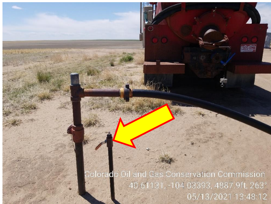
Photo 7 – Unmarked Riser at SE Corner Pit
