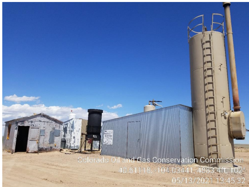
Photo 1 – Heater Treater, ECD, and Pump House
