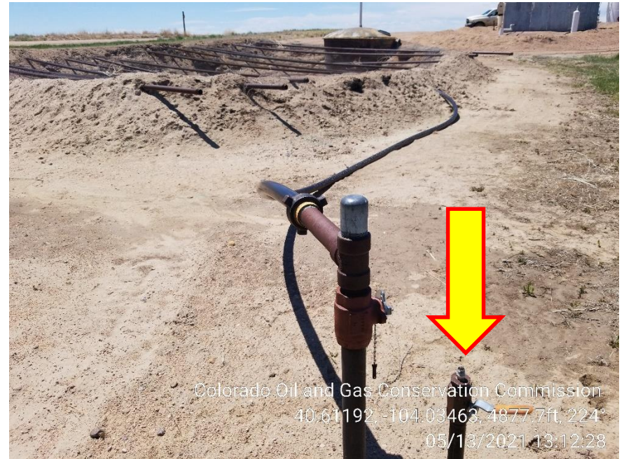
Photo 6 – Unmarked Risers at NE Corner of Pit
