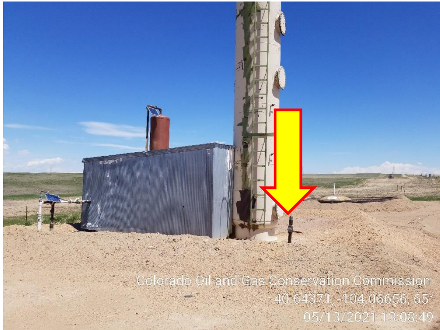
Photo 3 – Heater Treater, unmarked Riser
