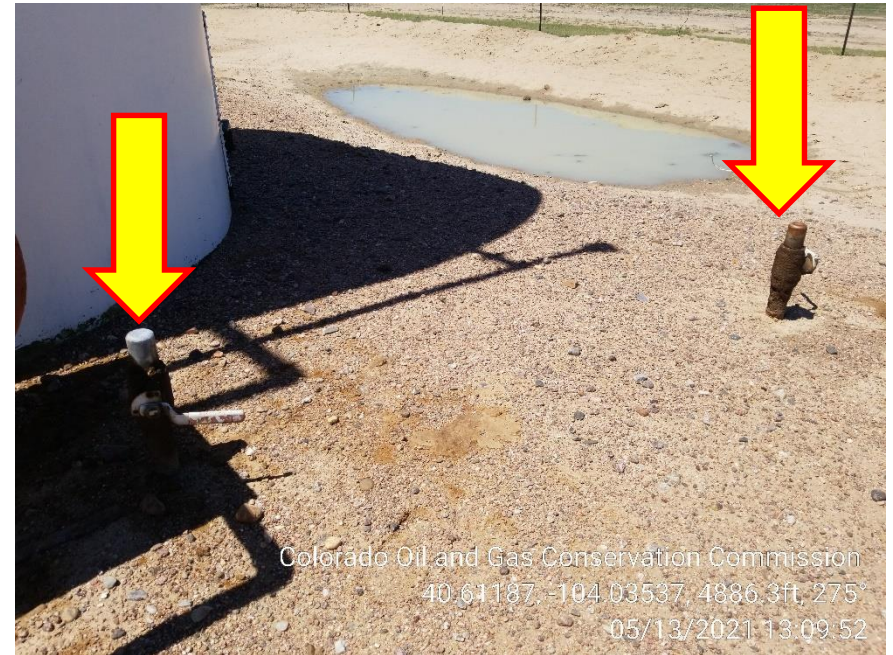
Photo 4 – Unmarked Risers at Tanks
