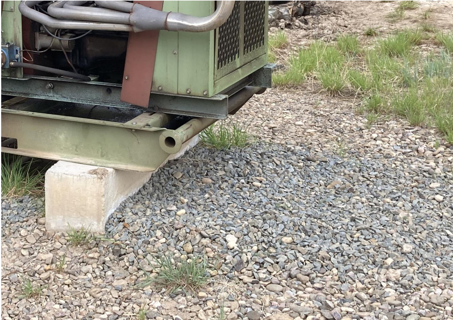
PHOTO 3: THE LEAKING MUFFLER ON THE ENGINE SKID WAS REPAIRED AND ALL FITTINGS WERE SECURLY FASTENED.
