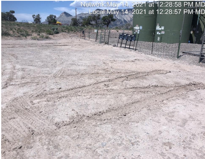
Photo #3813 location lacks stabilization.
