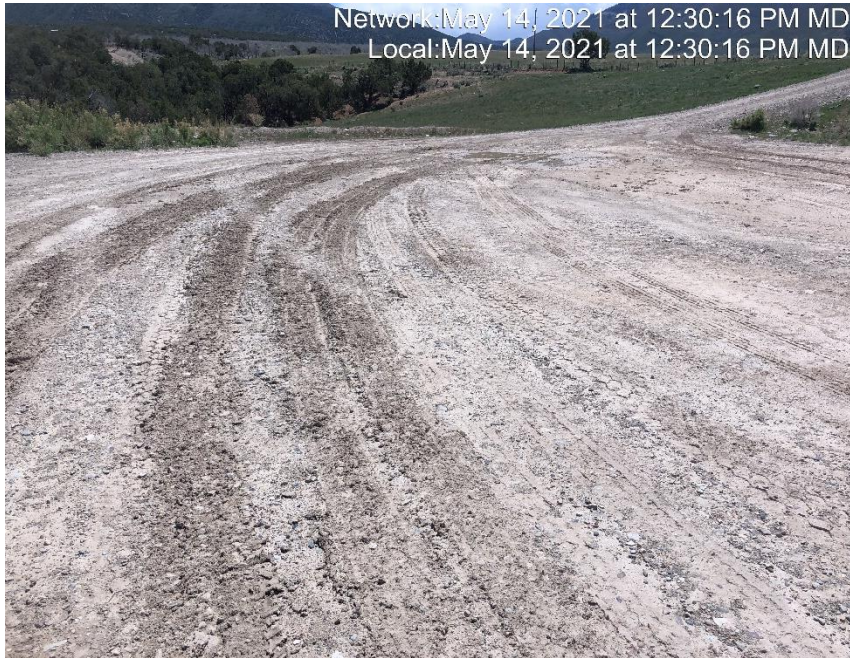
Photo #3815 No form of tracking BMP located at the entrance to location.
