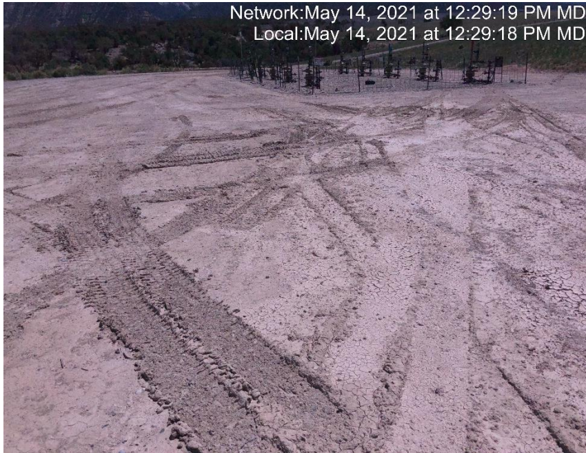
Photo #3814 Location lacks stabilization.
