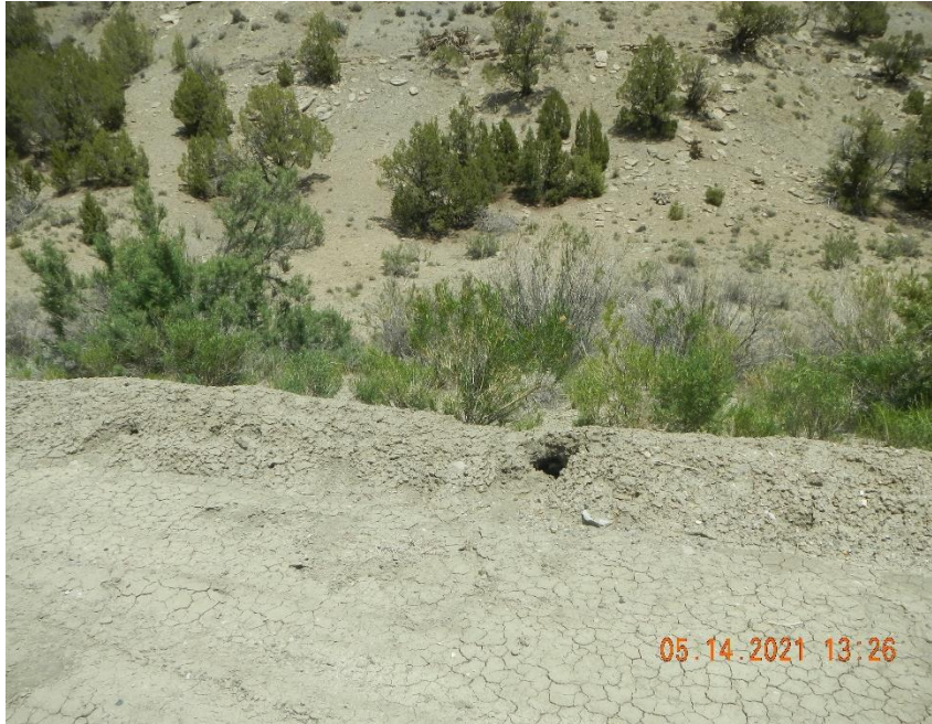
Channeling in perimeter berm.
