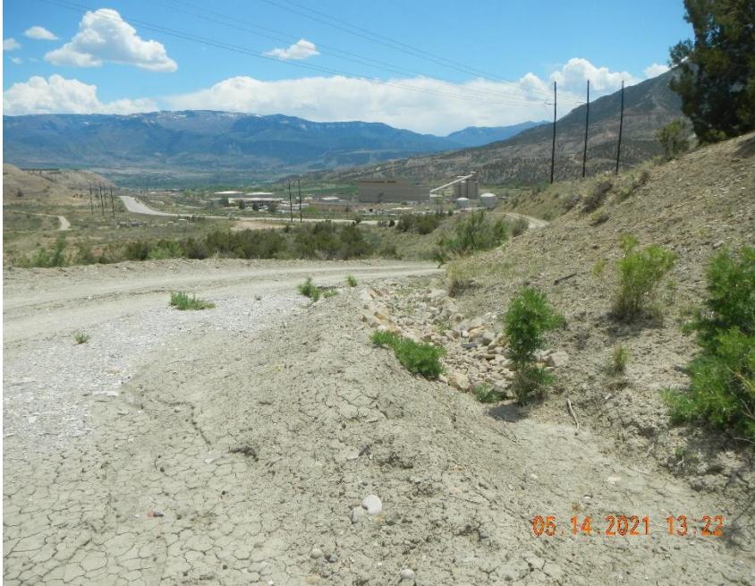
Riling along berm running to access road.
