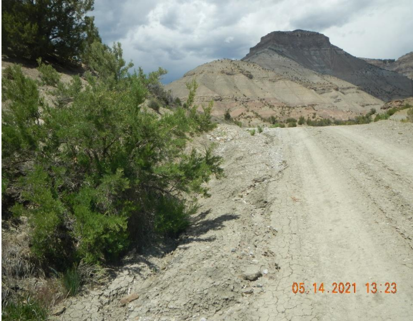
Riling from location running along ditch on access road.
