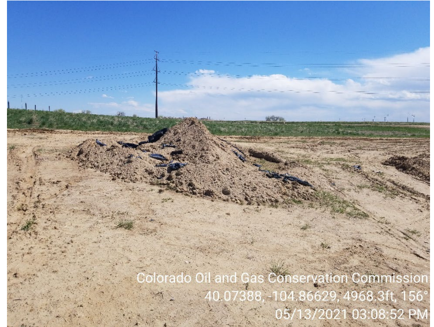
Photo 6 – Soils stockpiled on location. Lining does not adequately protect surface soils. BMPs inadequate for stormwater runoff.
