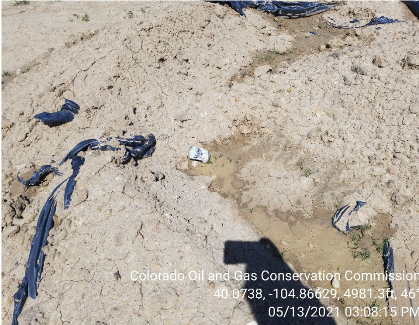
Photo 5 – Soils stockpiled on location. Lining does not adequately protect surface soils. Trash remains on location.
