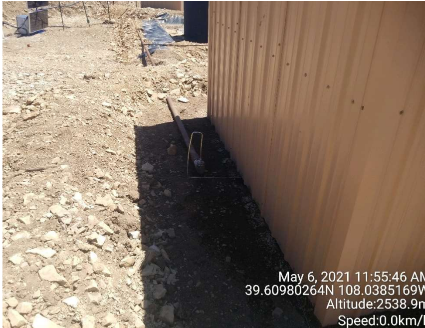
2-inch steel pipeline that is attached to the western structure via processing pipe.
