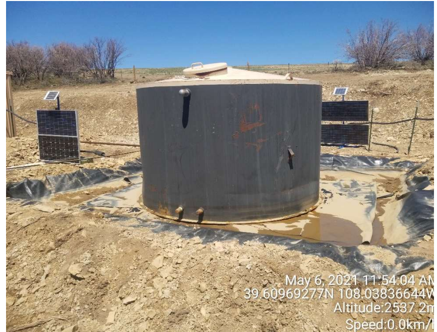
Steel AST inside a lined, earthen containment structure. Note the missing labels. Note the solar panels located next to multiple monitoring wells on location.
