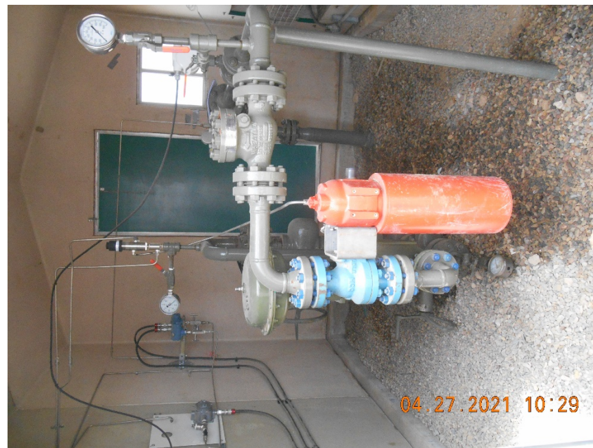
Injection well tubing gauge
