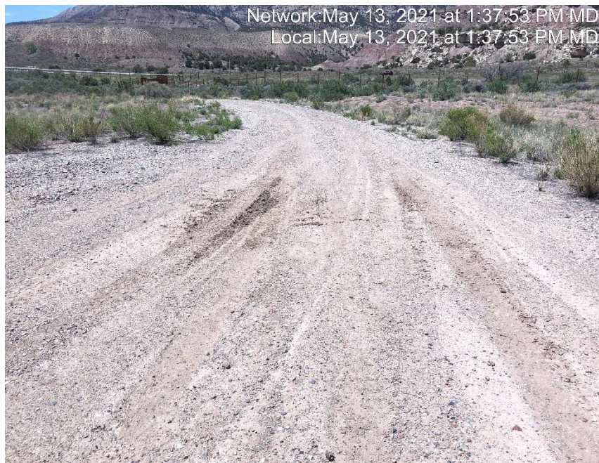
Photo #3804 No form of tracking BMP located at the entrance to location.
