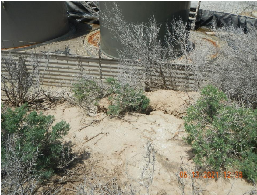
Erosion of bank behind tank battery.
