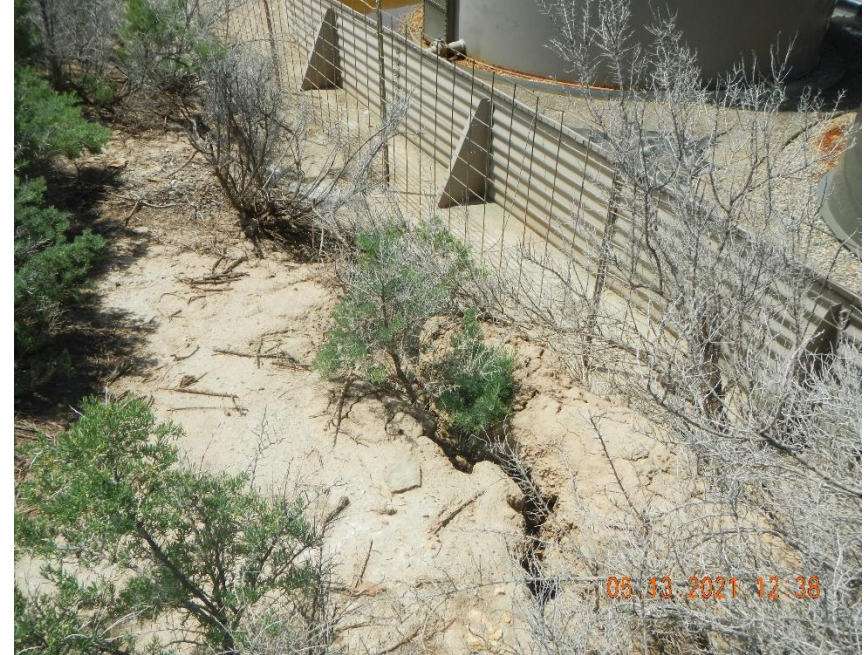
Erosion of bank behind tank battery.
