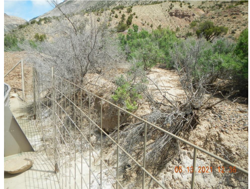
Erosion of bank behind tank battery.
