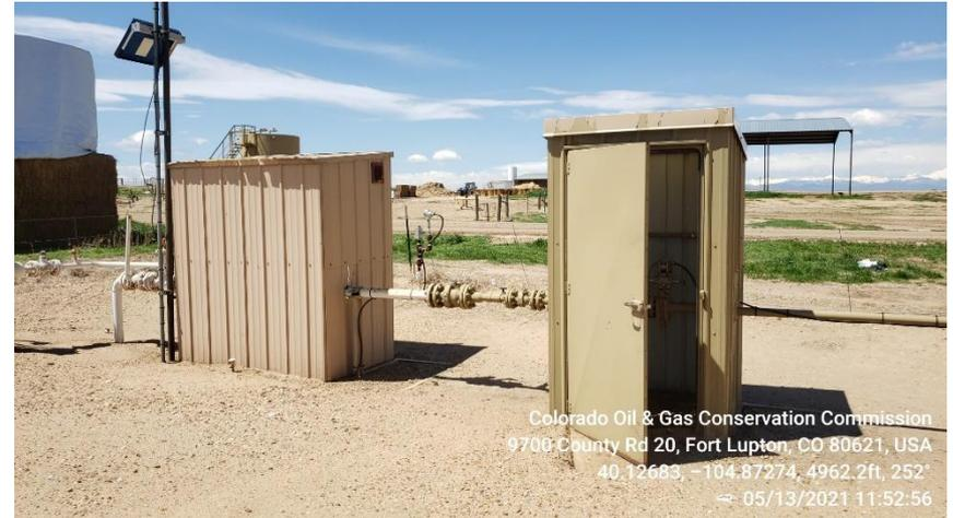
Photo 7 Horizontal Heated Separator
