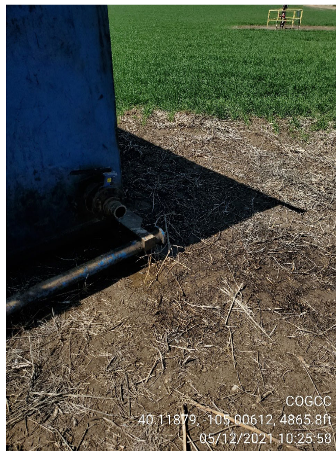
Photo 2 Leak from open top tank valve
