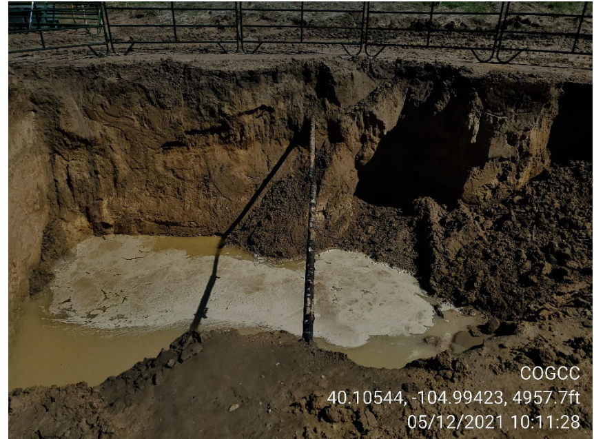
Photo 2 Excavation at flowline spill looking north
