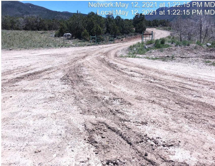
Photo #3788 No form of tracking BMP at entrance to location.
