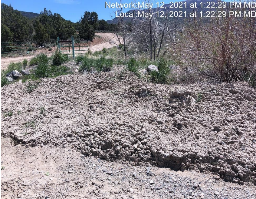
Photo #3789 Sediment has been transported off of location.
