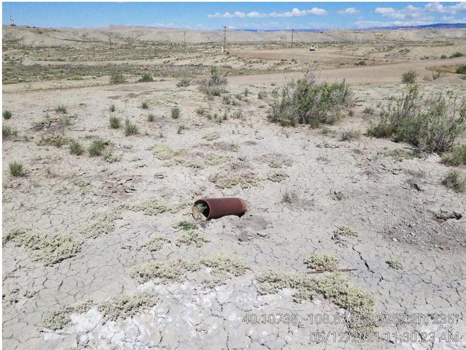
Photo 1. Location with pipe over open casing.
