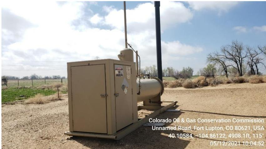
**Photo 9 Horizontal Heated Separator**
