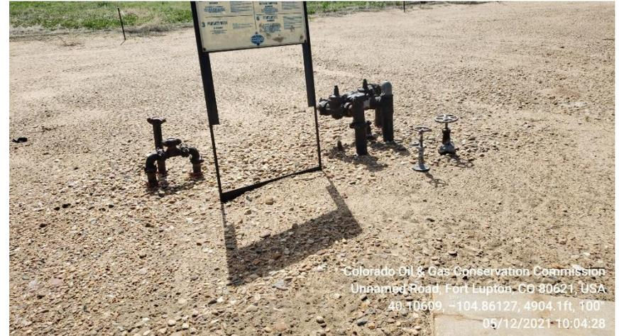
**Photo 7 Gas Meter Run No indication of calibration.**
