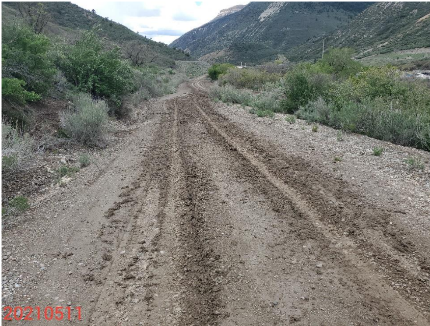
Photo 11: Photo taken from the access road, facing southwest. Photo shows BMPs to stabilize production areas/access road and to prevent off-location sediment transport during wet conditions are missing or insufficient
