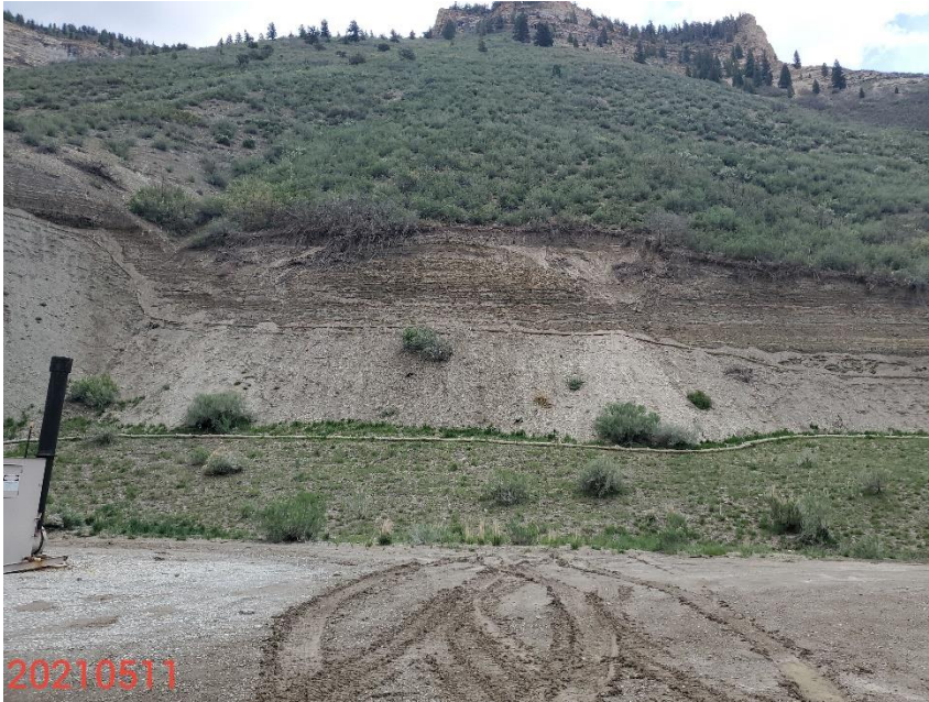
Photo 7: Photo taken from the production area, facing east. Operator has installed wattles along the base and upper portions of the cut slope; no other control measures were observed to be used in conjunction with the wattles on the slopes. Photo shows areas where erosion on the cut slopes have covered multiple sections of wattles. BMPs to stabilize/protect remain missing or insufficient.
