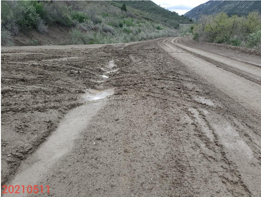
Photo 13: Photo taken from the access road entrance, facing south. Photo shows BMPs to stabilize production areas/access road and to prevent off-location sediment transport during wet conditions are missing or insufficient
