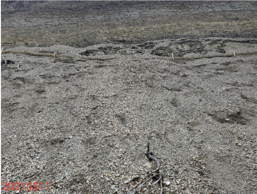
Photo 9: Photo shows areas where erosion on the cut slopes have covered multiple sections of wattles.
