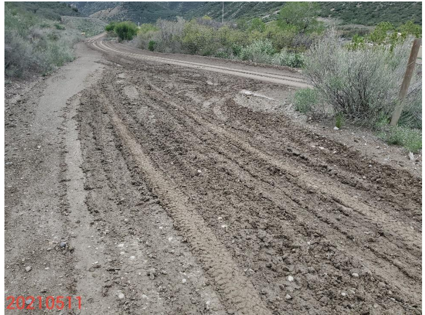
Photo 12: Photo taken from the access road entrance, facing southwest. Photo shows BMPs to stabilize production areas/access road and to prevent off-location sediment transport during wet conditions are missing or insufficient
