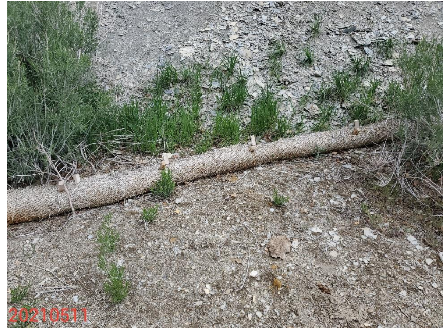
Photo 8: Photo shows wattles along base of cut slope; wattles do not appear to have been properly trenched and backfilled in accordance with good engineering practices.
