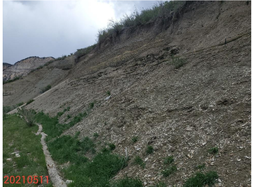
Photo 10: Photo taken from the cut slope on the east end of the Location, facing north. Operator has installed wattles along the base and upper portions of the cut slope; no other control measures were observed to be used in conjunction with the wattles on the slopes. BMPs to stabilize/protect remain missing or insufficient.
