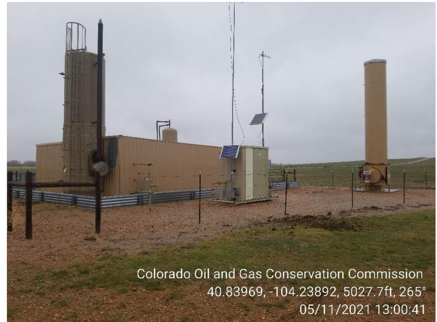
Photo 4 – Treater, Gas Meter and ECD
