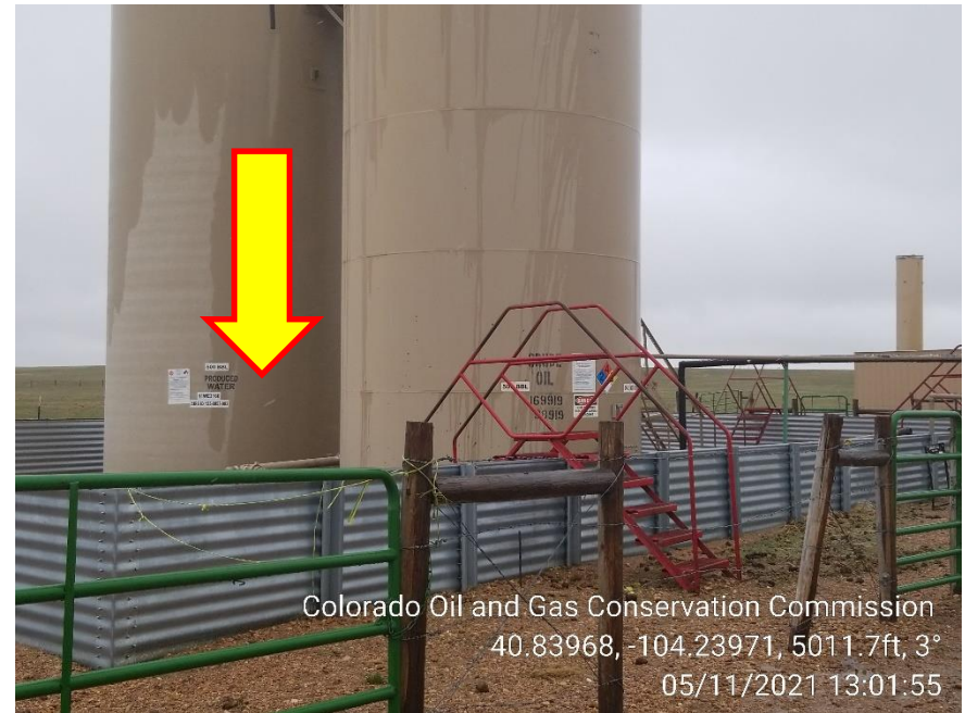
Photo 6 – Tank Battery - H2O Tank missing NFPA Label
