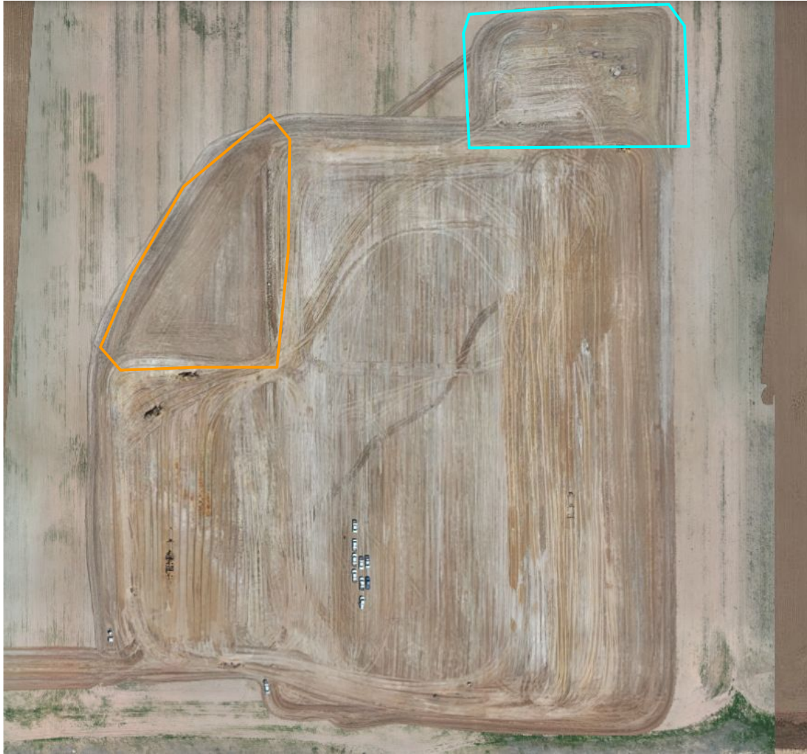
Photo 1. Drone aerial imagery taken during construction operations. Photo illustrates the topsoil stockpile (orange) and the detention pond (blue).
