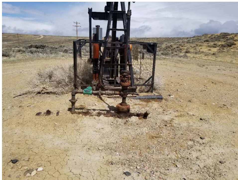
Photo 1. No bradenhead access apparent.
