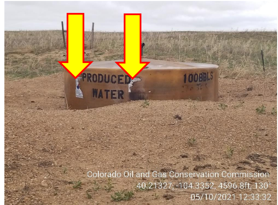
Photo 4 – Produced Water Tank – NFPA Label Weathered
