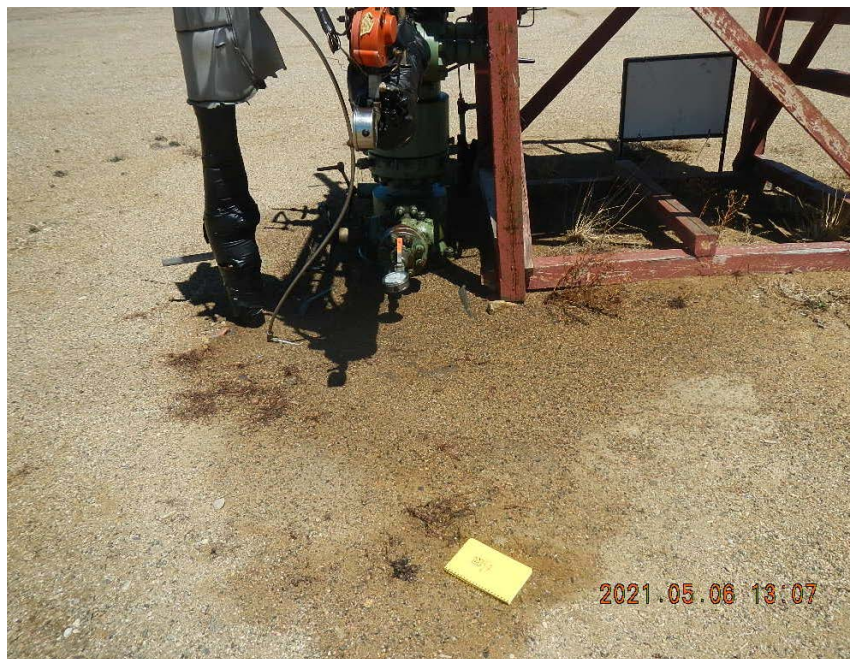
Staining from on-going gas leak/vent and condensate around wellhead.
