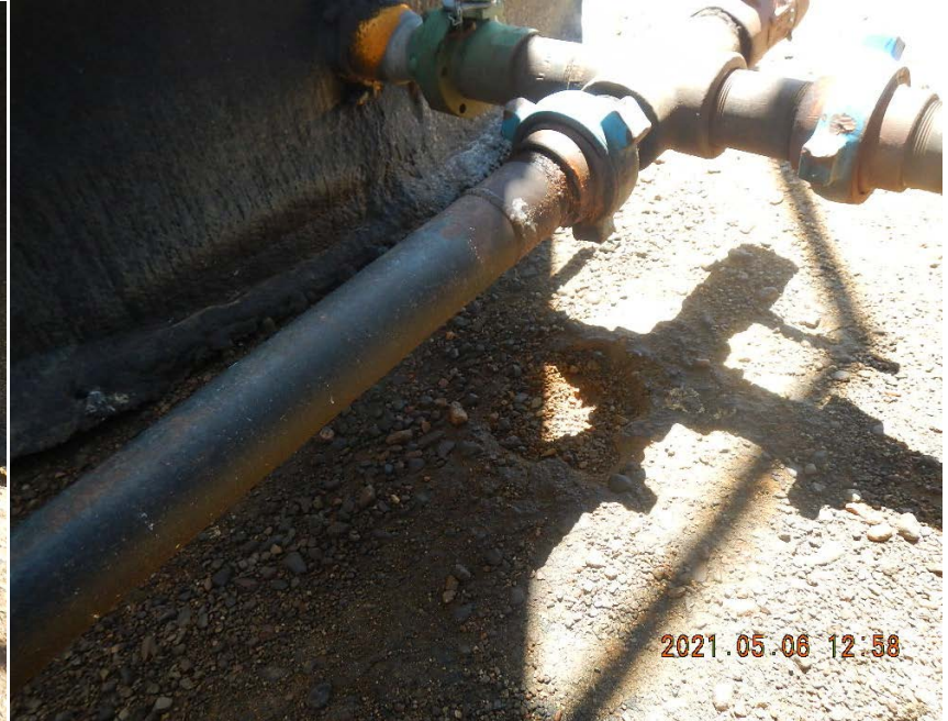
Tank 0030, staining beneath hammer unions.
