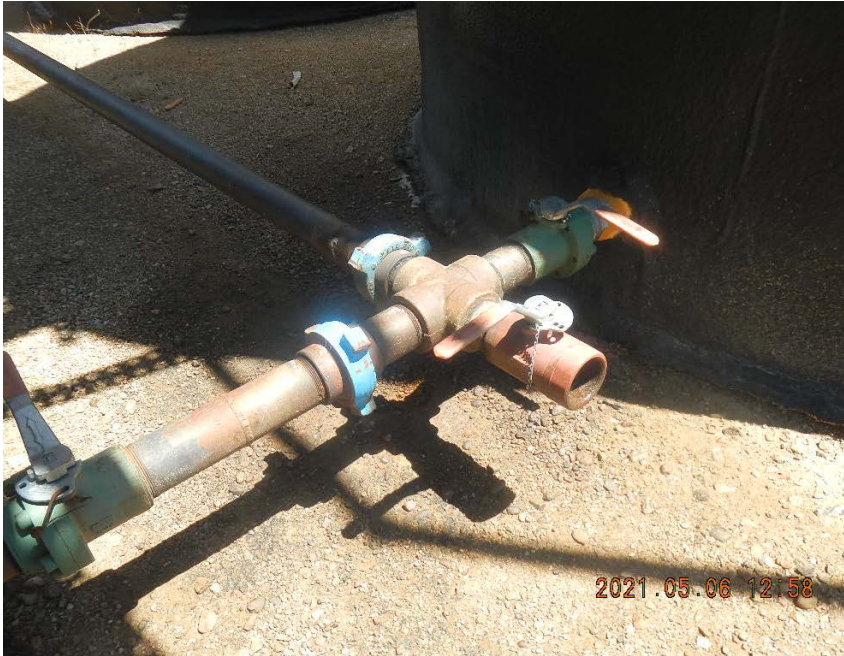
Tank 0030, staining beneath hammer unions.
