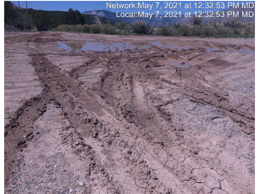
Photo #3754 Location lacks stabilization.
