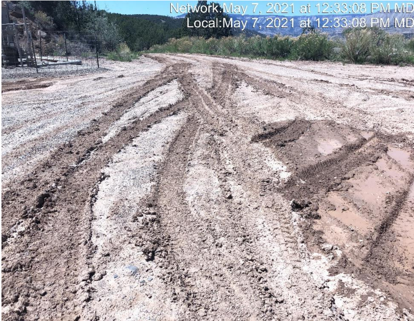
Photo #3755 No form tracking BMP located at entrance to location.
