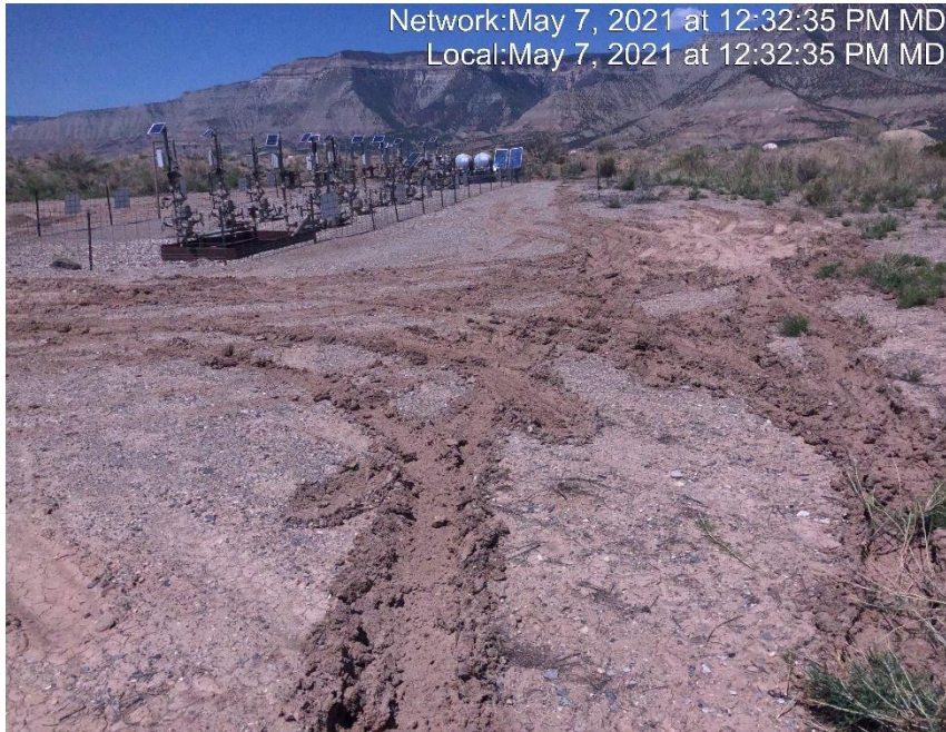
Photo #3753 Location lacks stabilization.
