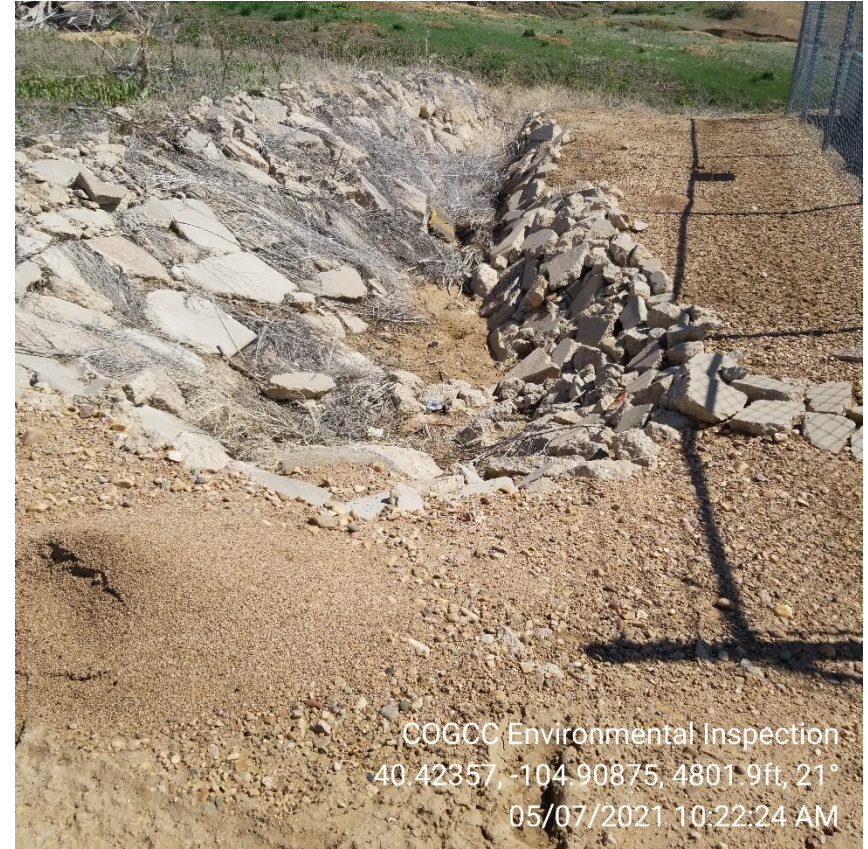
Photo 6 – Outfall of stormwater diversion.
