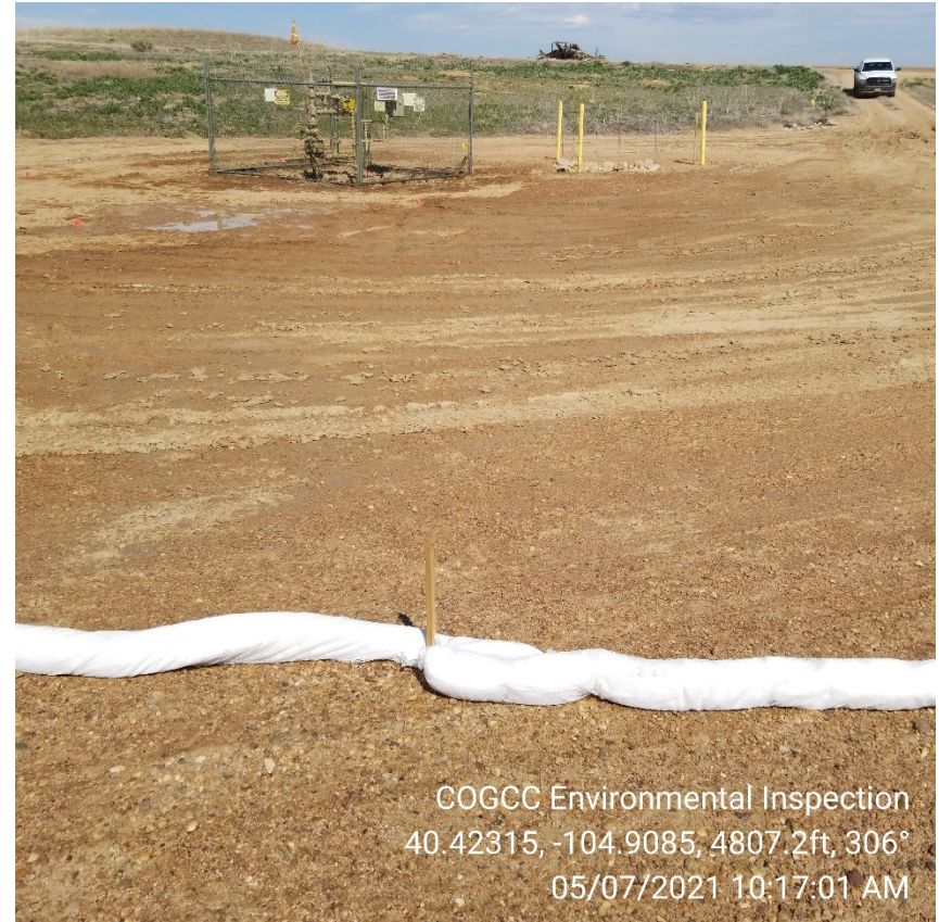
Photo 4 – Absorbent booms placed on downhill area of pad.
