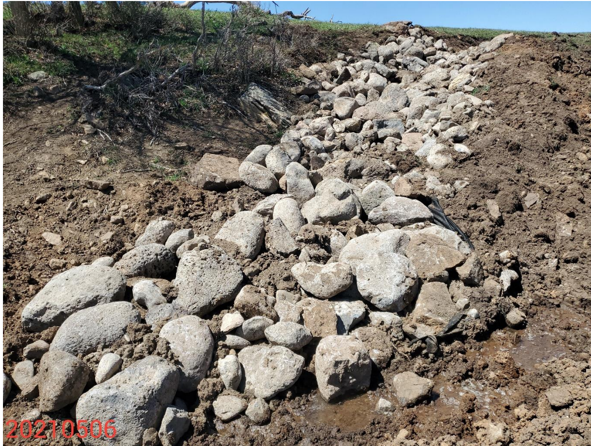
Photo 9: Photo taken from the northwest corner of the Location, facing north. Photo shows Operator has installed armoring along section of the ditch that travels downslope. Rock used is very large and not properly sized per good engineering practices. Geotextile lining has been placed beneath the riprap.
