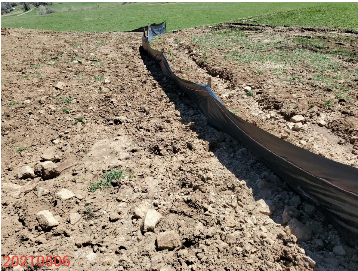
Photo 11: Photo taken from the southwest end of the Location, facing east. Photo shows Operator has installed silt fence as a temporary measure to manage runoff.
