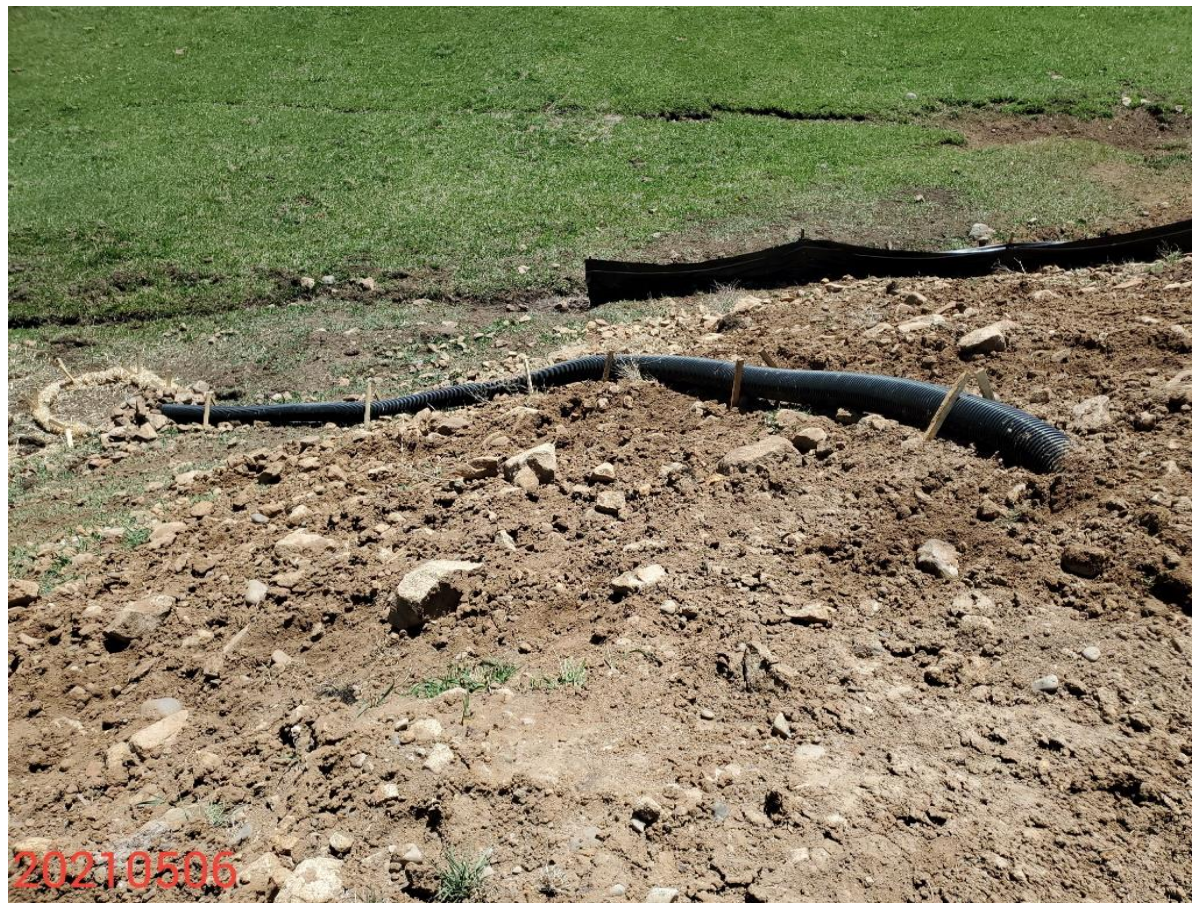
Photo 15: Continued from photo 13. Photo shows slope drain and the outlet. Unclear if the slope drain is sufficiently secured.
