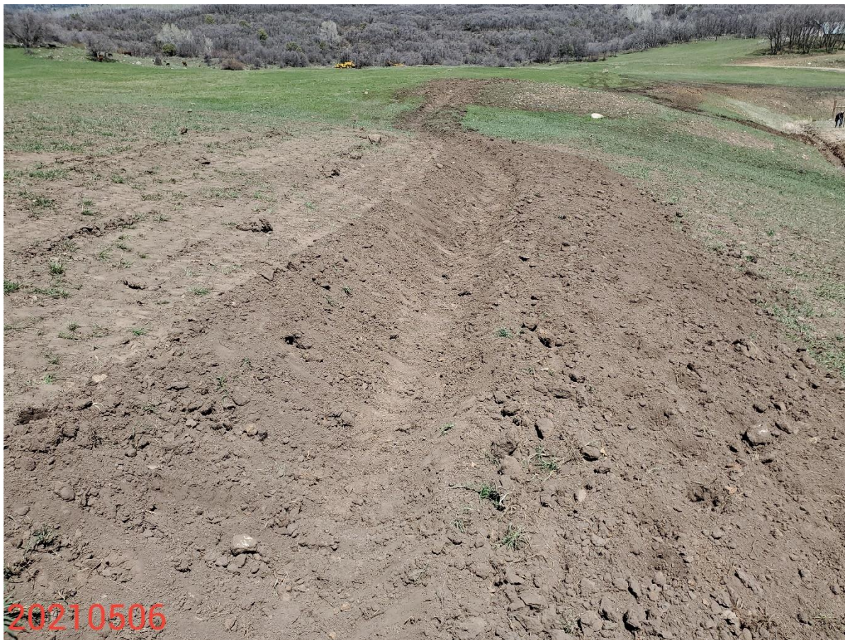
Photo 6: Photo taken from the north of the Location, facing east. Construction activities to address stormwater issues observed to be in process at time of inspection. Photo shows ditch being constructed to manage runoff.
