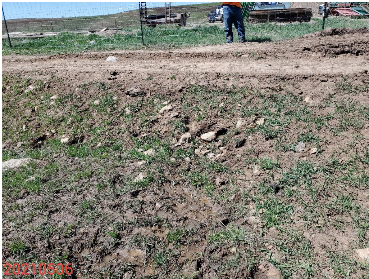
Photo 18: Photo taken from the south end of the Location. Operator has installed a drain/culvert that travels beneath the soils from the pad to the slopes. Drain has not been constructed with an appropriate outlet.
