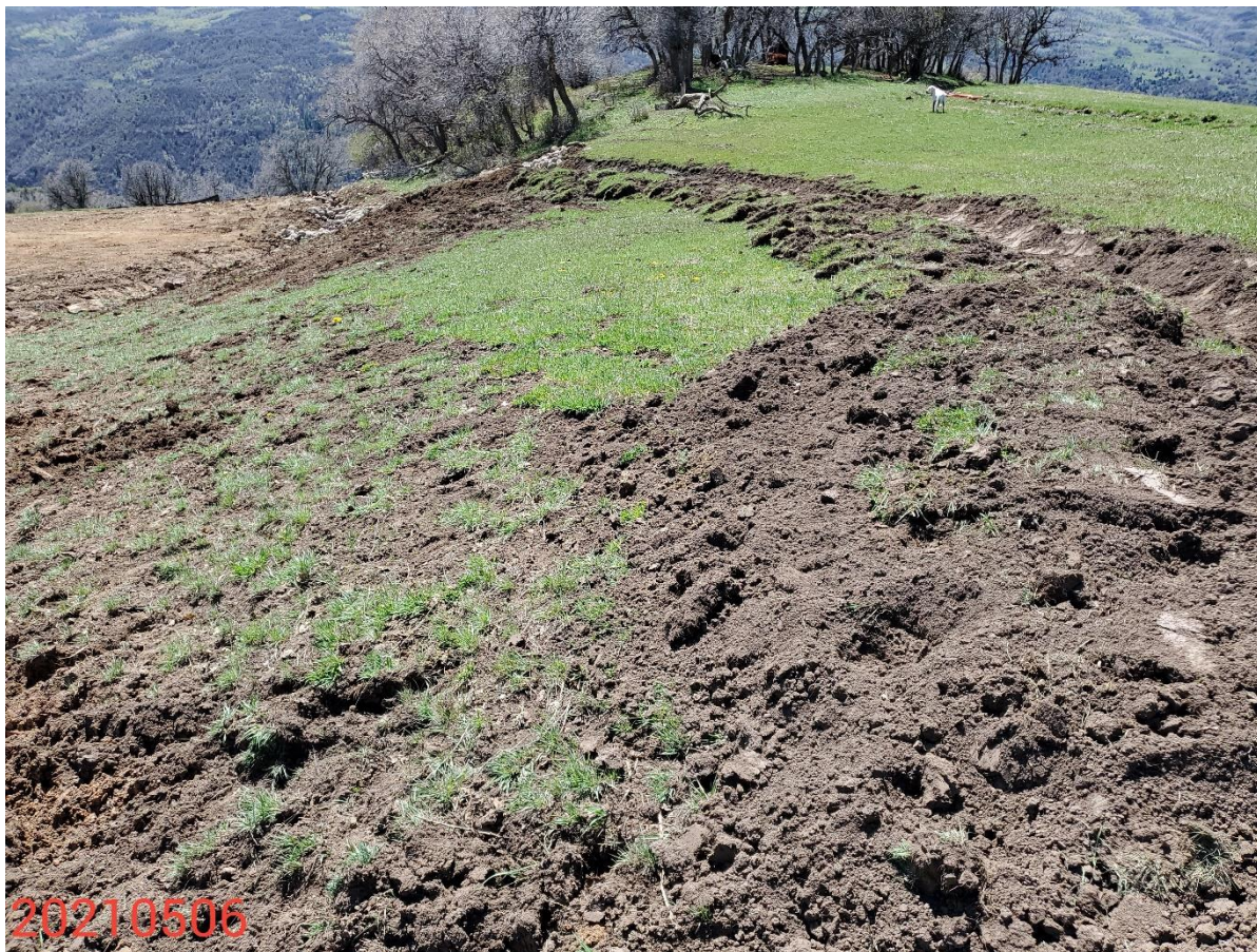
Photo 7: Photo taken from the north of the Location, facing west. Construction activities to address stormwater issues observed to be in process at time of inspection. Photo shows ditch being constructed to manage runoff.
