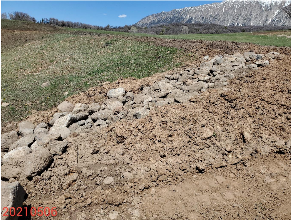
Photo 1: Photo taken from the east end of the Location, facing north. Construction activities to address stormwater issues observed to be in process at time of inspection. Photo shows ditch and armoring in process of being constructed to manage runoff. Armoring has been constructed with different sized aggregate and lined with geotextile.
