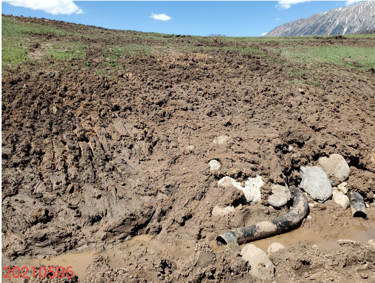
Photo 4: Photo taken from the cut slopes on the north end of the Location. Photo shows the sloughing slope observed in previous inspections has been repaired and a French drain system has been install. Slopes still requiring stabilization control measures and revegetation.
