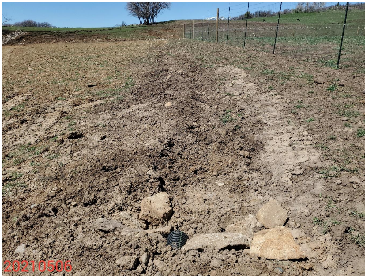
Photo 13: Photo taken from the ditch on the west end of the former pad, facing north. Photo shows inlet to a slope drain that has been installed at end of the Ditch.
