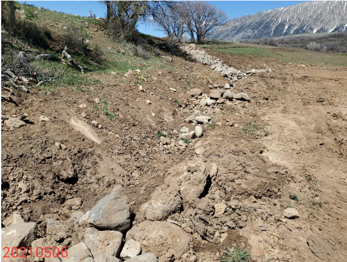
Photo 10: Photo taken from the west end of the Location, facing northeast. Construction activities to address stormwater issues observed to be in process at time of inspection. Operator on site indicated control measures such as a sediment trap or pond is being considered at the end of the ditches to allow for appropriate stormwater discharge from the disturbance area.
