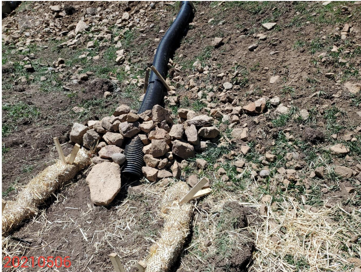
Photo 16: Continued from photo 13. Photo shows slope drain has not been constructed with an appropriate outlet in accordance with good engineering practices.
