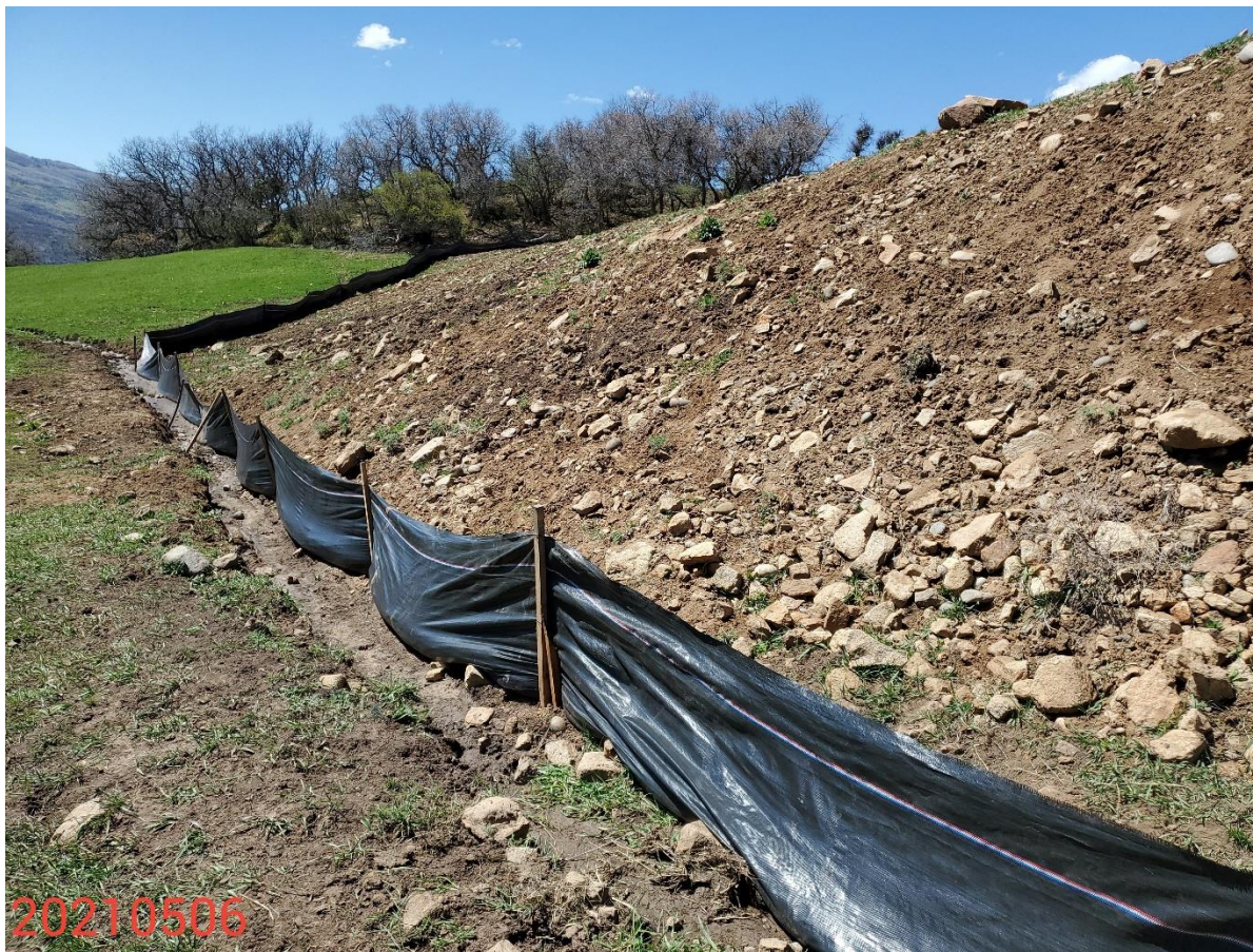
Photo 17: Photo shows silt fence along the western areas of the Location's disturbance.
