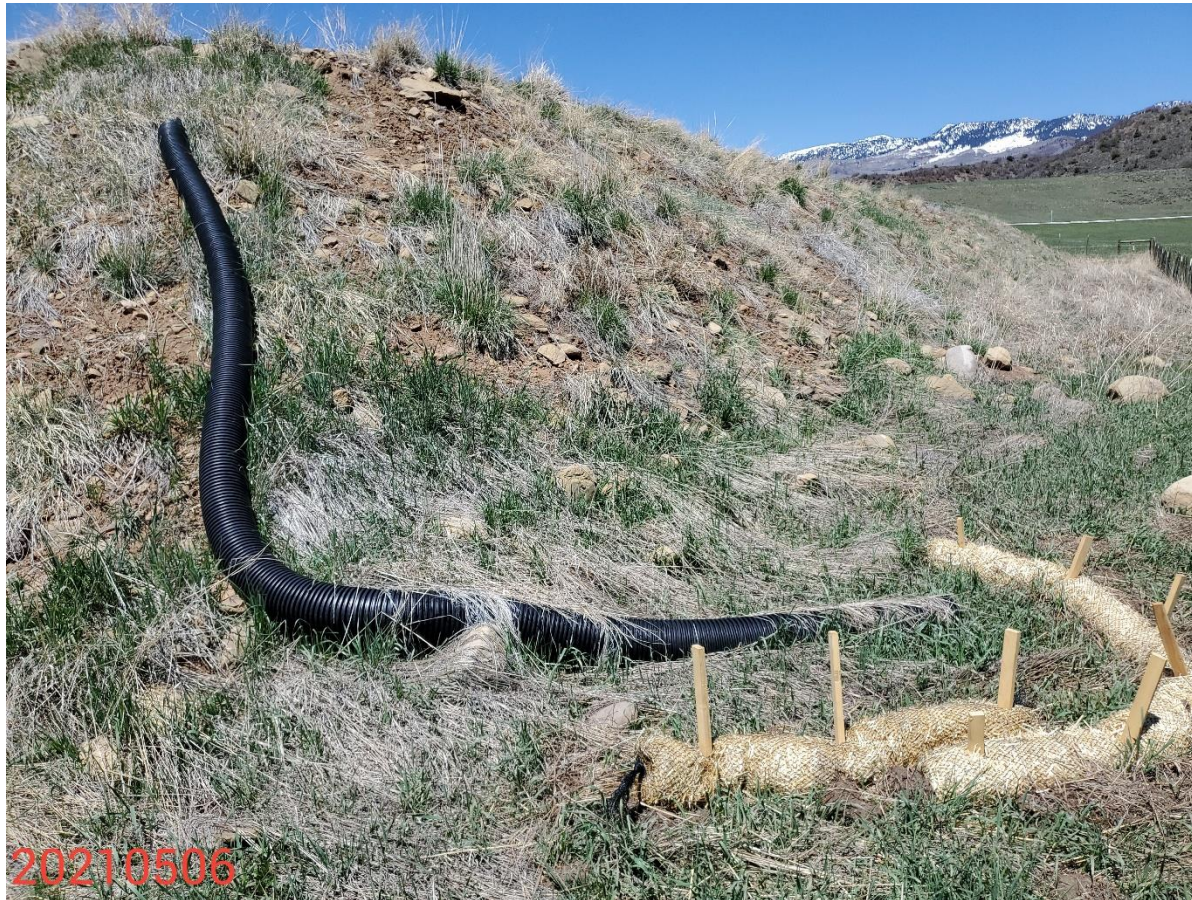
Photo 10: Photo taken from the southwest corner of the Location. Photo shows slope drain. Previous inspections documented that the slope drain was not been constructed with an appropriate outlet per good engineering practices. Photo shows slope drain has not been constructed with an appropriate outlet. Photo also shows slope drain has not been properly secured.
