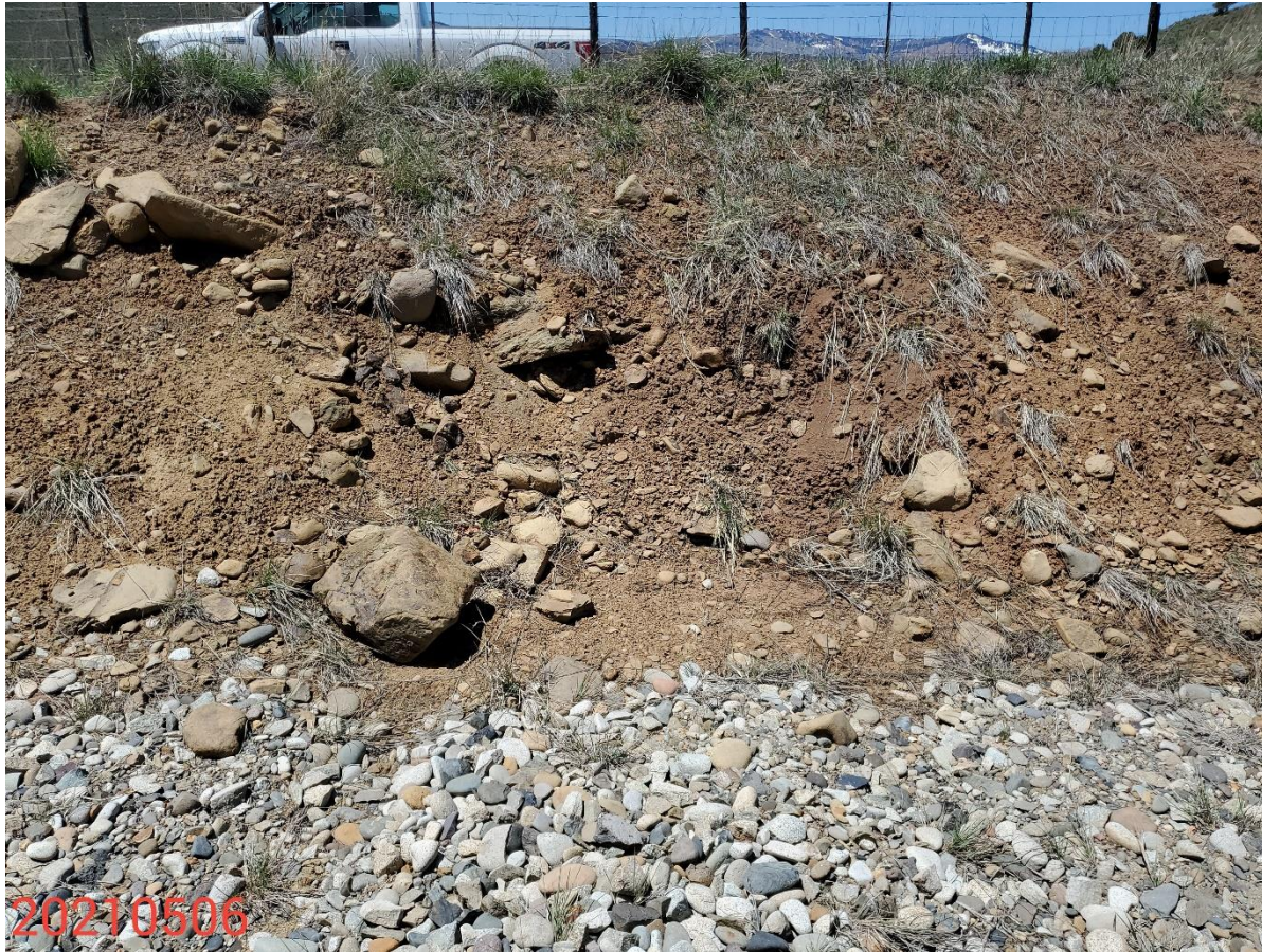
Photo 2: Photo taken from the cut slopes on the north end of the Location, facing north. Previous inspections documented that control measures to protect/stabilize slopes on the Location were missing or insufficient. Photo shows control measures to protect/stabilize slopes on the Location remain missing or insufficient.
