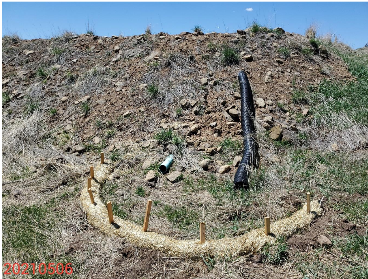
Photo 8: Photo taken from the southeast corner of the Location. Photo shows slope drain. Previous inspections documented that the slope drain was not been constructed with an appropriate outlet per good engineering practices. Photo shows slope drain has not been constructed with an appropriate outlet. Photo also shows slope drain has not been properly secured.
