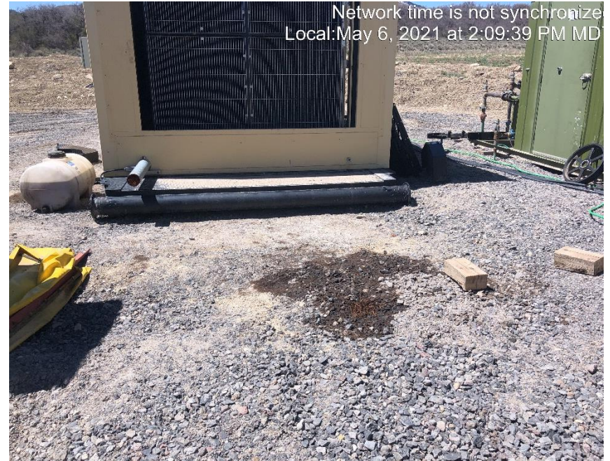
Photo #3749 Multiple places with stained soil outside of containment.
