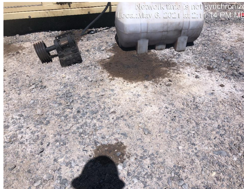
Photo #3750 No chemical BMP located at chemical tank. Stained soils under chemical tank.
