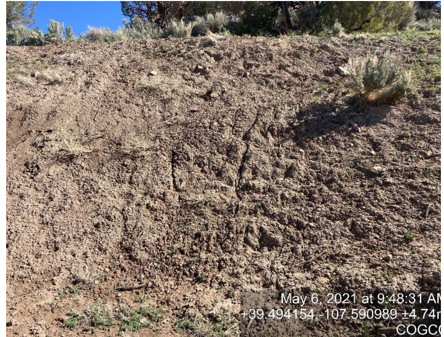
Cut slope lack of stabilization/erosion photo from follow up inspection
