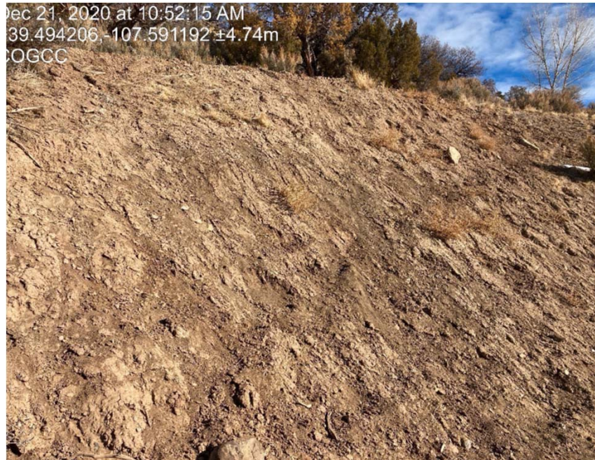
Cut slope lack of stabilization/erosion photo from previous inspection
