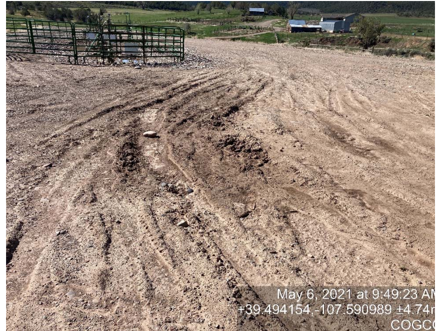
Lack of stabilization/compaction
