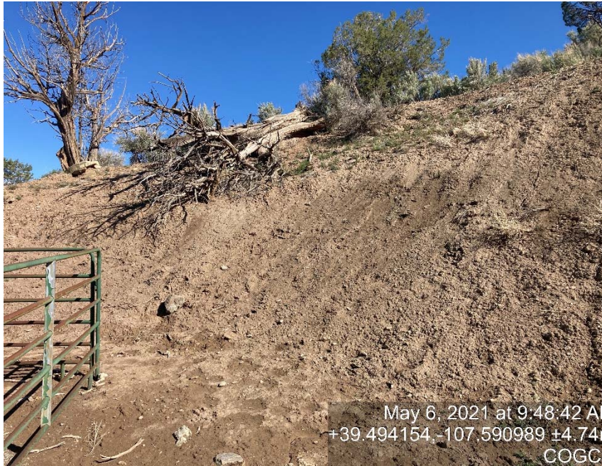
Cut slope lack of stabilization/erosion
