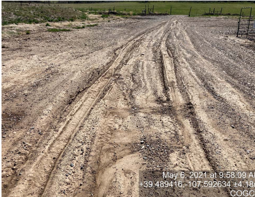
Lack of stabilization/compaction
