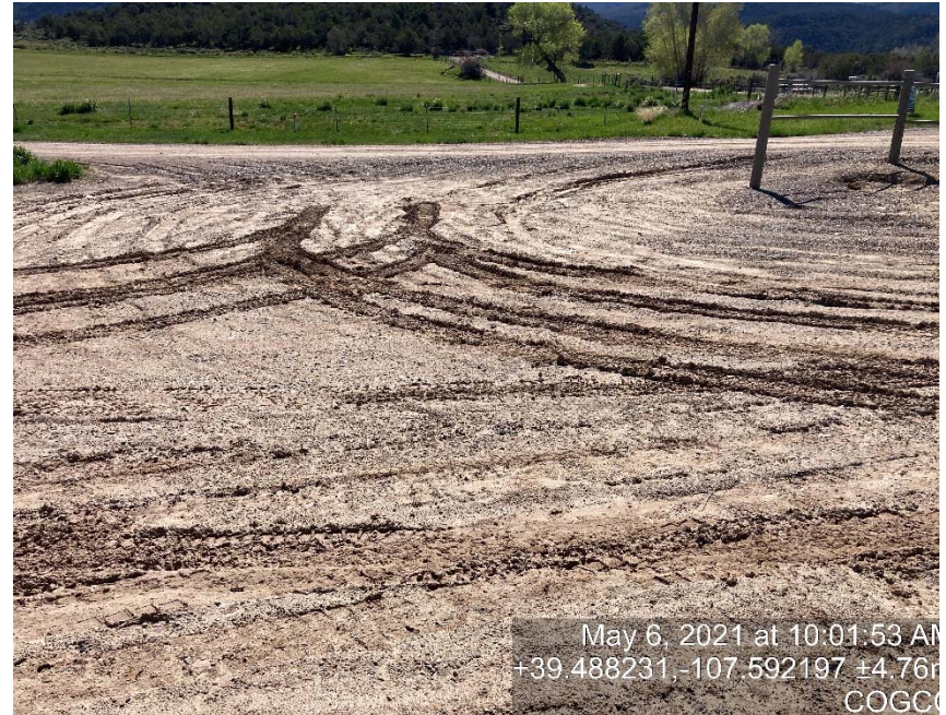
Lack of stabilization/compaction
