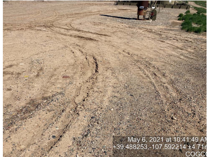
Lack of stabilization/compaction
