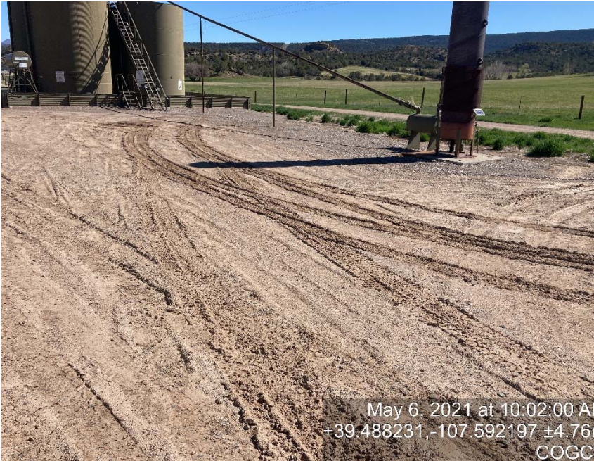
Lack of stabilization/compaction
