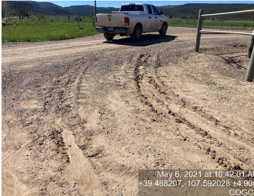
Lack of stabilization/compaction
