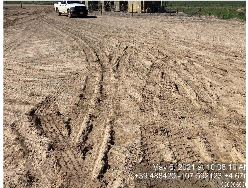
Lack of stabilization/compaction
