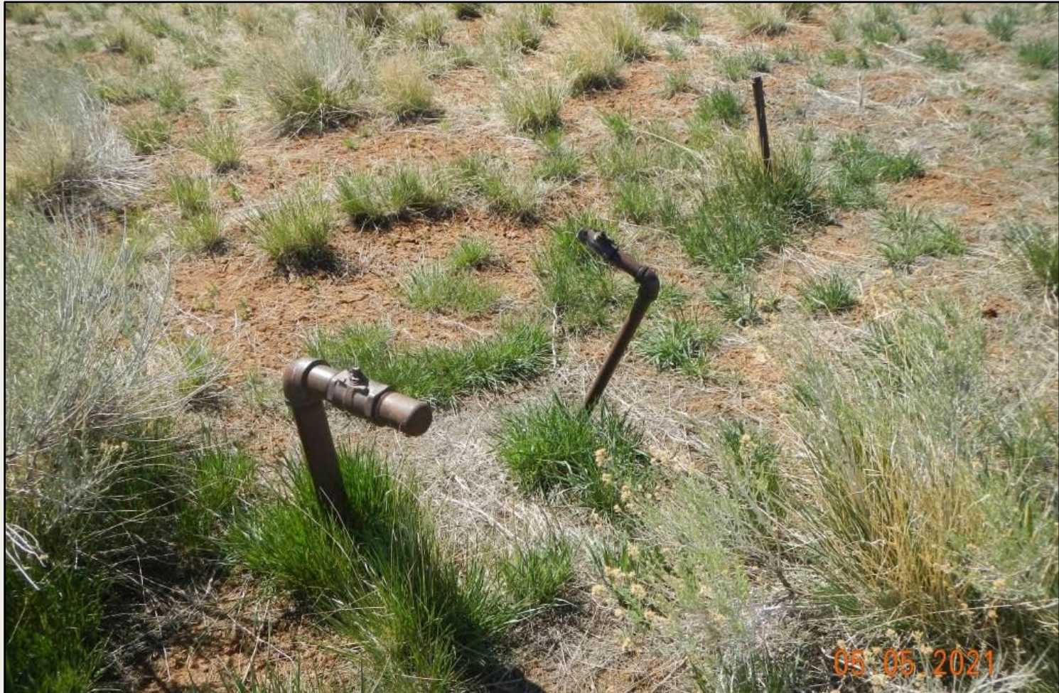
Photo 3. View of risers that remain within the northeastern project area, need to be properly abandoned and removed.
