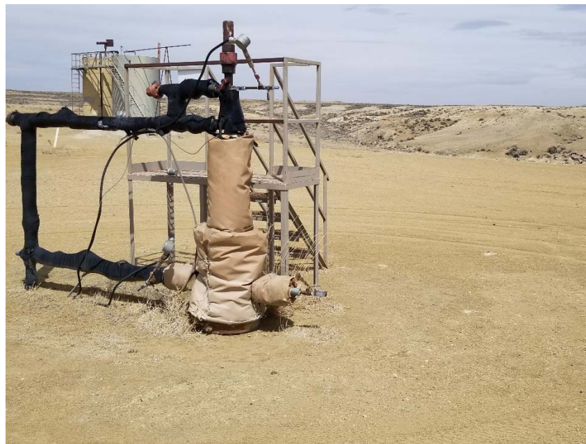
Photo 2. No bradenhead access apparent.
