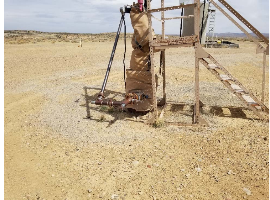
Photo 2. No bradenhead access apparent.
