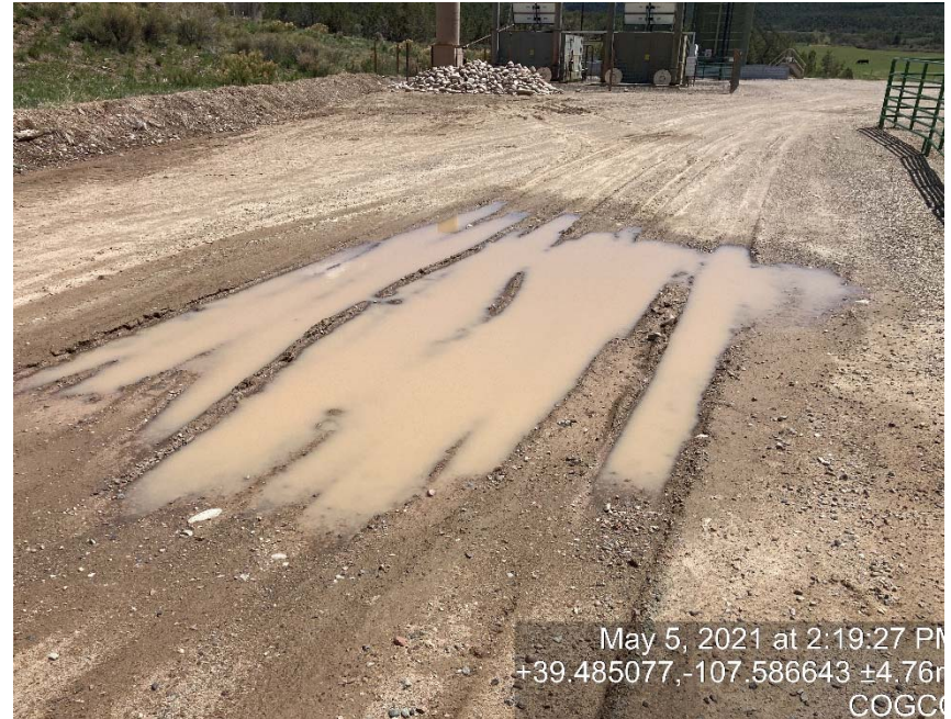
Lack of stabilization/compaction
