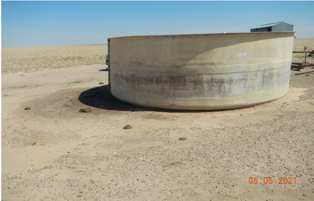
Photo 5. Secondary containment is inadequate to contain 150% of the volume of the tank.
