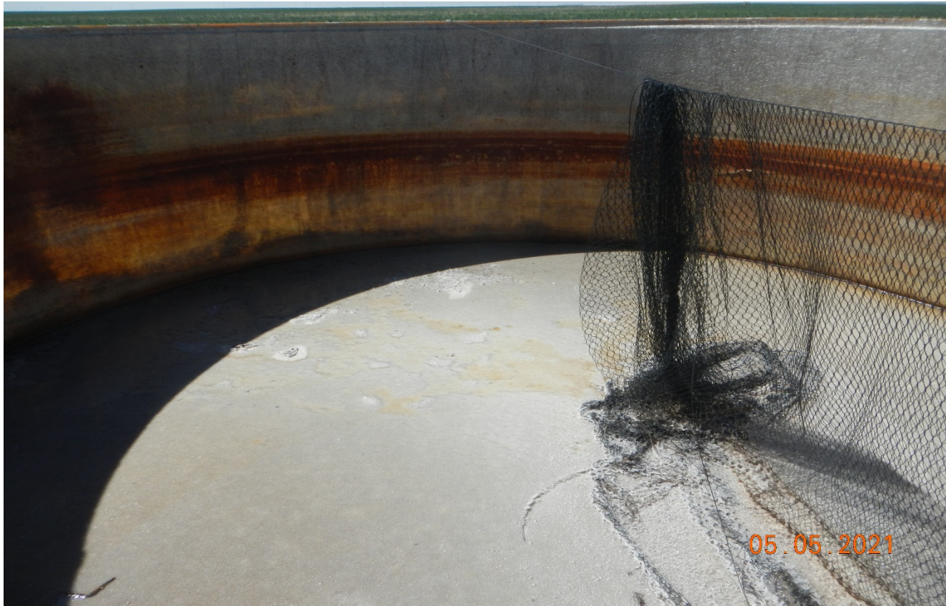
Photo 5. View of fluids inside the tank. Tank is labeled Produced Water. It appears to be solidified salty produced water. The netting on the tank is in disrepair.
