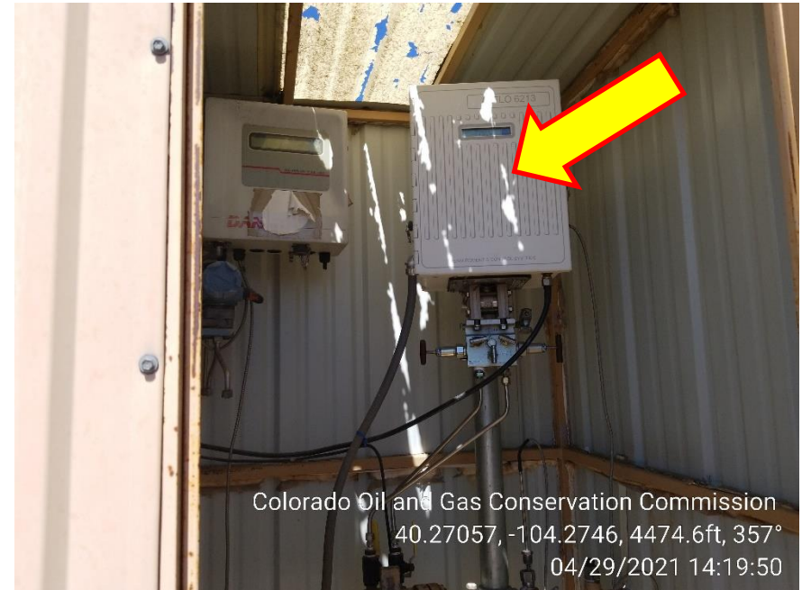
Photo 12 – Gas Meter Calibration Card missing
