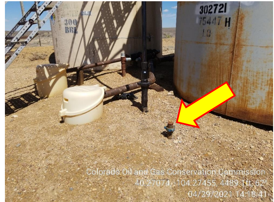
Photo 10 – Unmarked Risers
