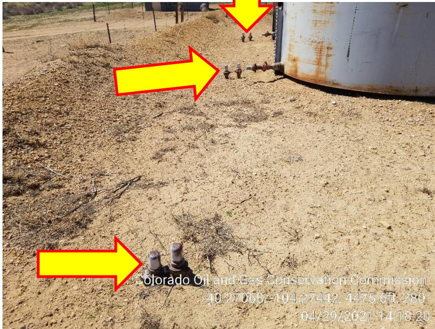
Photo 9 – Unmarked Risers
