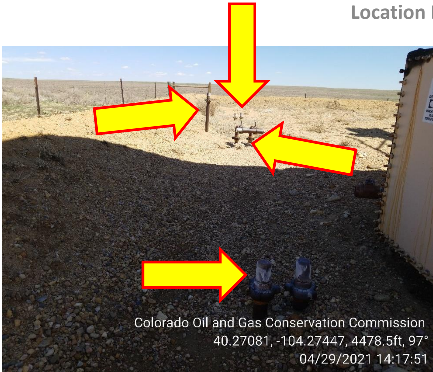
Photo 7 – Unmarked Risers
