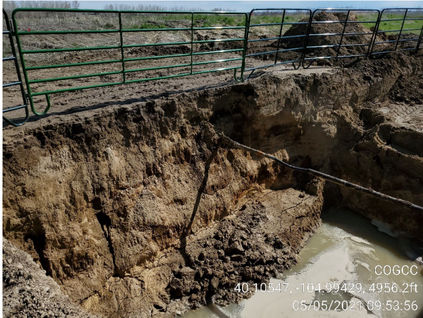
Photo 3 Excavation at flowline Spill, looking northeast
