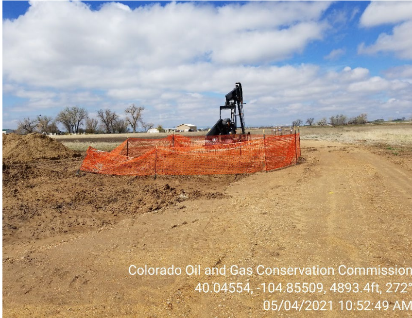
Photo 1 – Spill area. Fencing repaired around open excavation.
