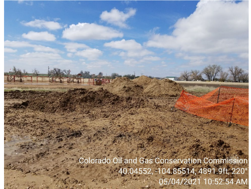
Photo 4 – Soil stored on location with inadequate BMPs.
