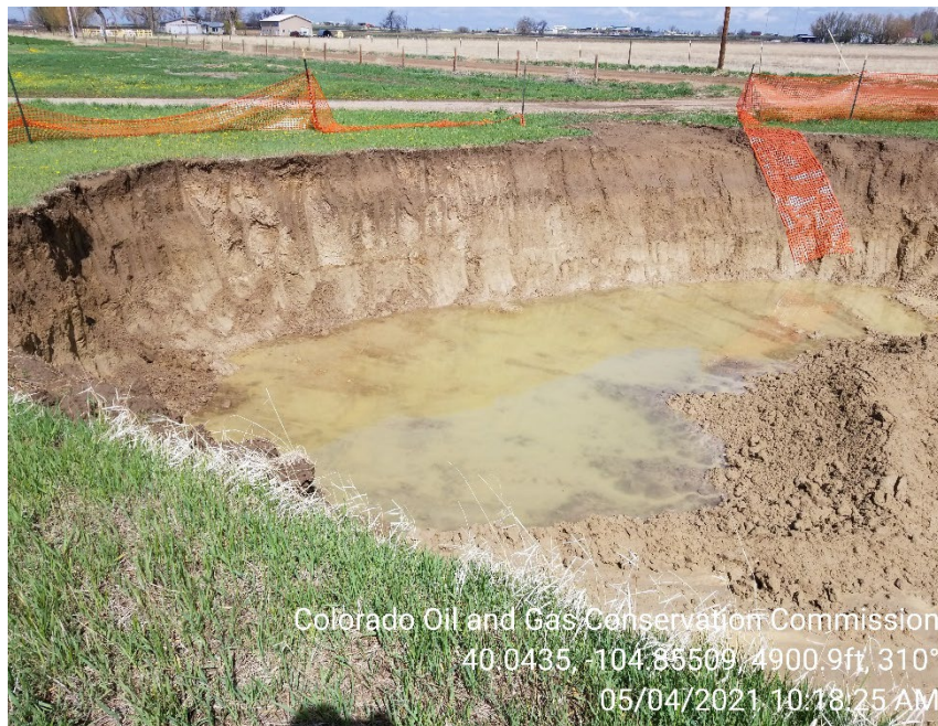
Photo 5 – Spill excavation. Impacts appear to remain in situ. Groundwater observed in open excavation.
