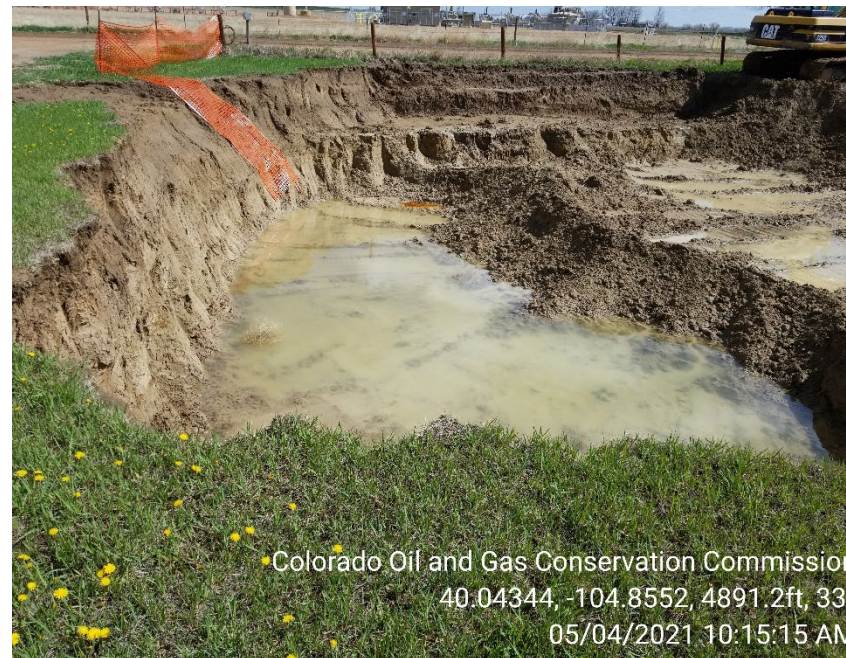
Photo 2 – Spill excavation. Impacts appear to remain in situ. Groundwater observed in open excavation.
