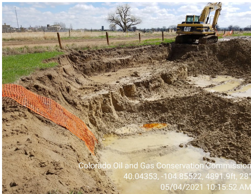
Photo 3 – Spill excavation. Impacts appear to remain in situ. Groundwater observed in open excavation.
