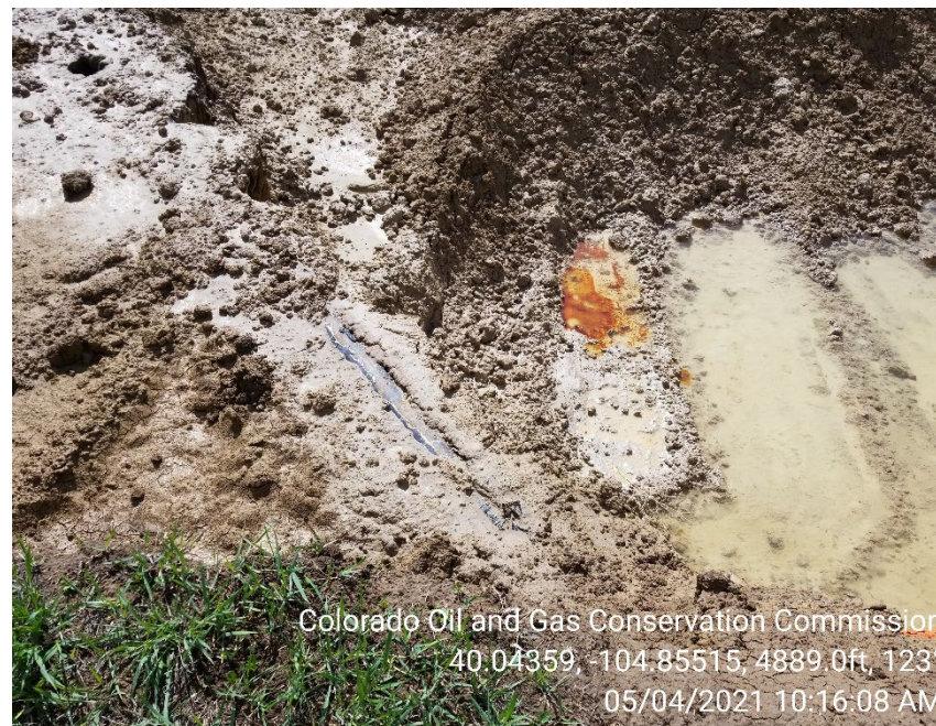
Photo 4 – Exposed flowline in open excavation.
