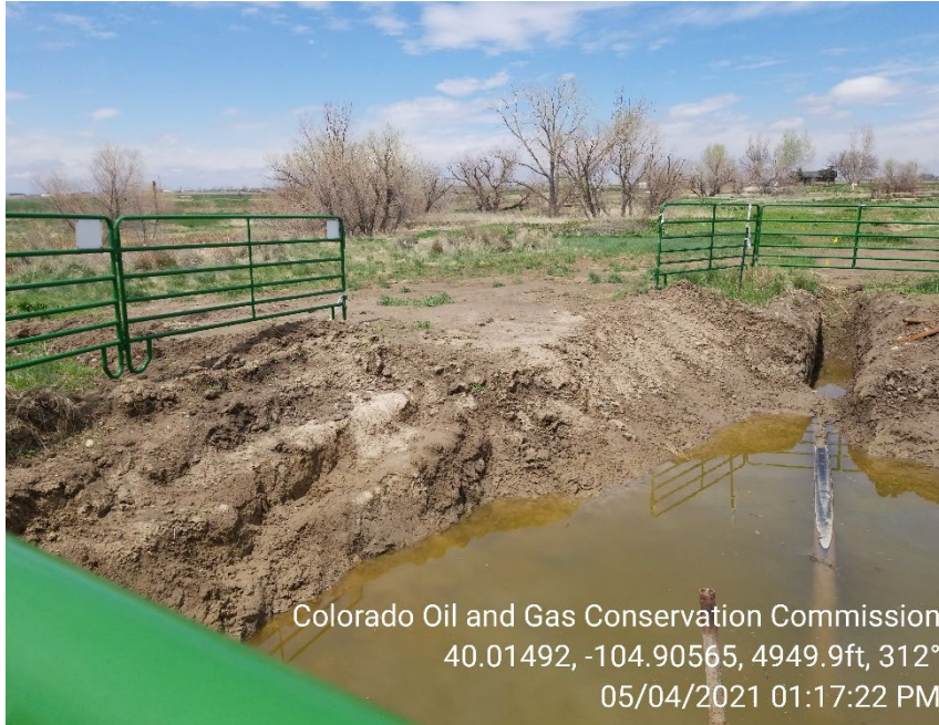
Photo 3 – Fencing around open excavation does not adequately protect access to the site.
