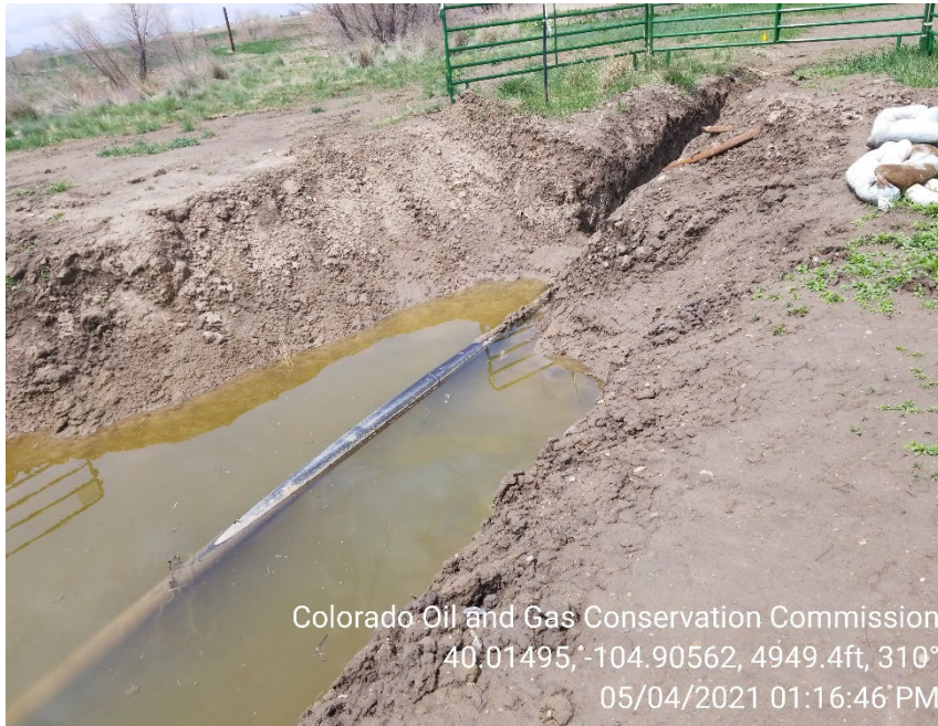
Photo 5 –Open excavation. Hydrocarbon sheen observed on groundwater.
