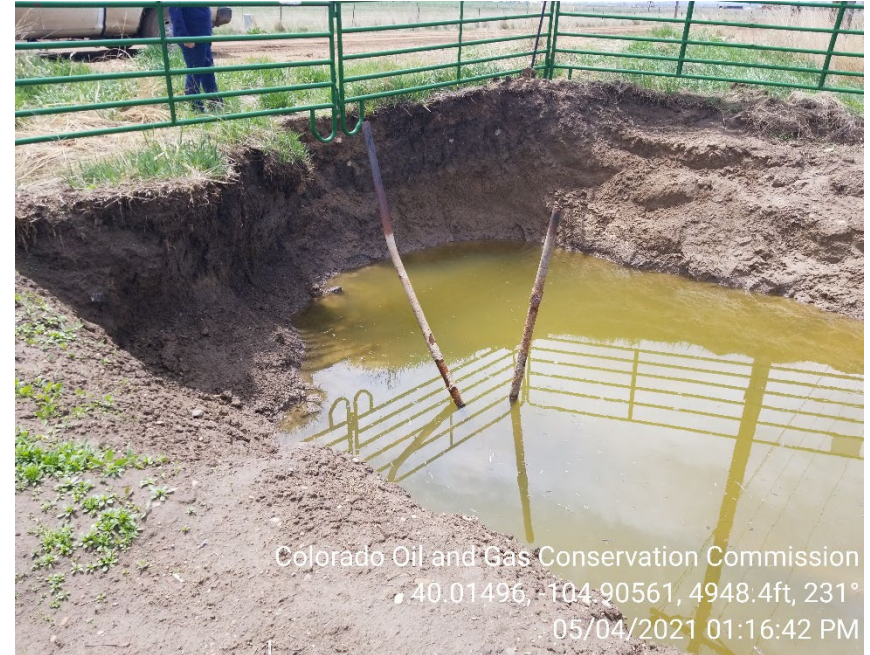
Photo 4 – Open excavation. Impacts appear to remain in situ. Hydrocarbon sheen observed on groundwater.
