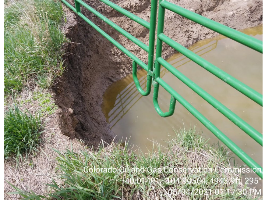
Photo 2 – Fencing around open excavation does not adequately protect access to the site.
