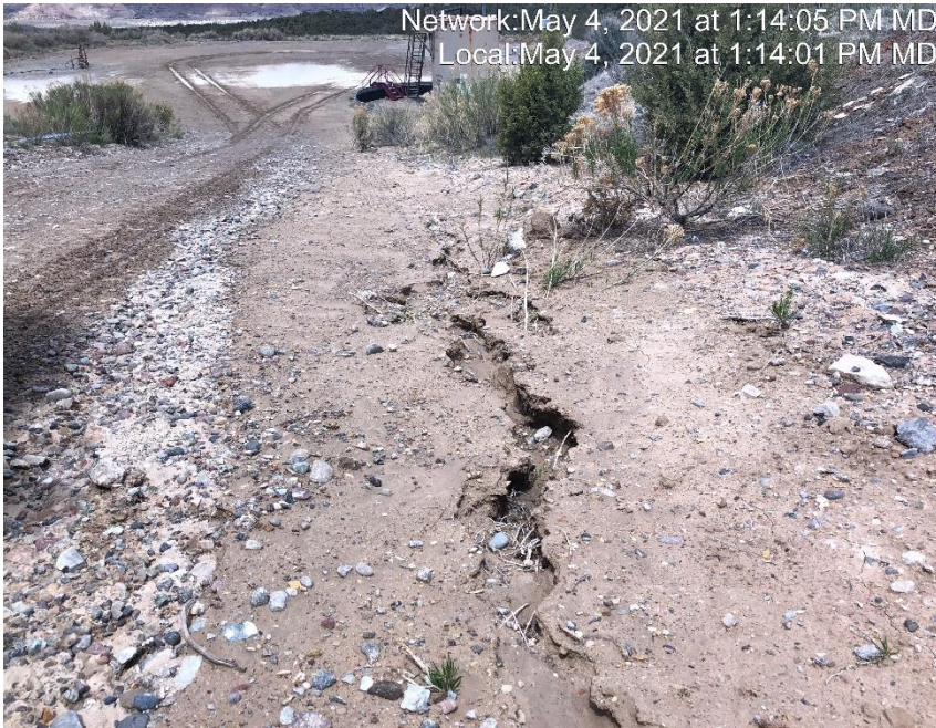
Photo #3695 Run on to location is not being controlled.
