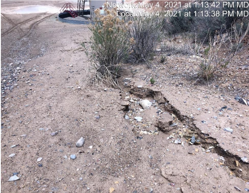
Photo #3694 Gully erosion occurring on Eastside of access road.
