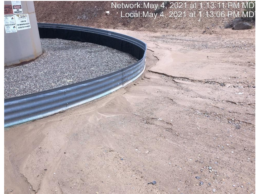
Photo #3693 Sediment is encroaching on tank containment.
