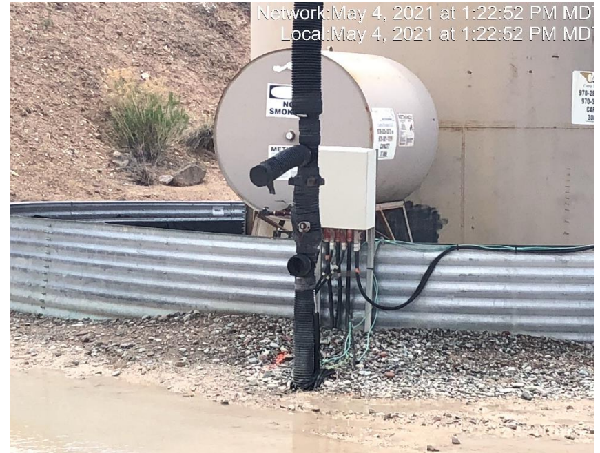
Photo #3697 Heating insulation open ended and not capped.
