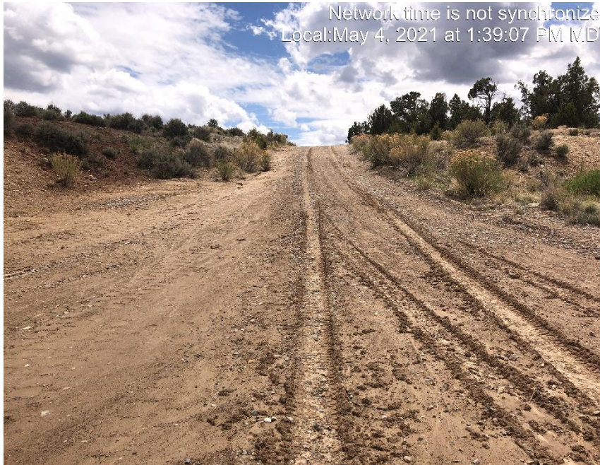
Photo #3698 no form of tracking control at entrance to location.
