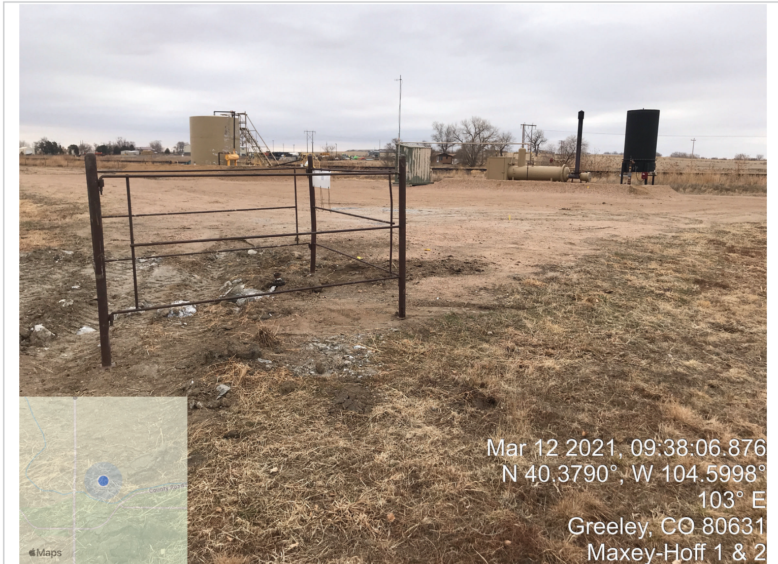
Photo Point D: Facility Pad - Facing Southeast From Northwest Perimeter
