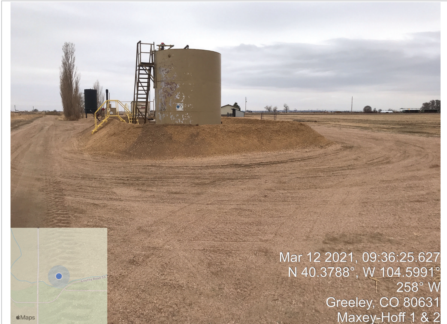
Photo Point A: Facility Pad - Facing West From Southeast Corner
