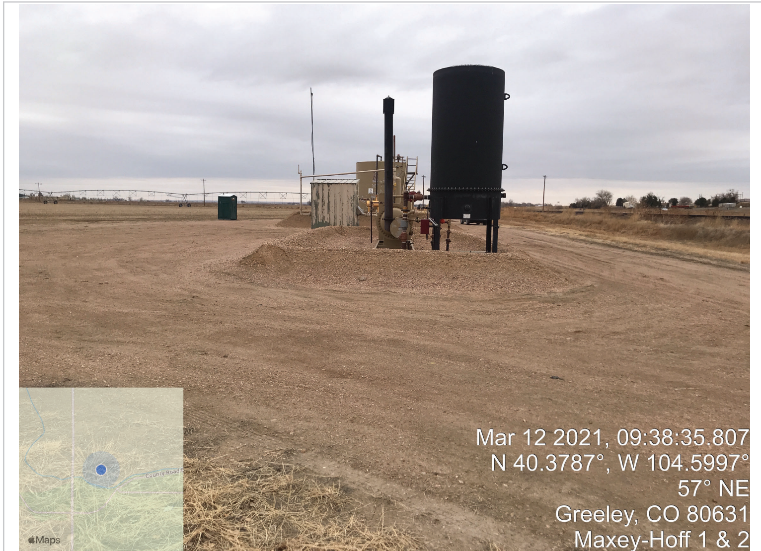
Photo Point C: Facility Pad - Facing Northeast From Southwest Perimeter
