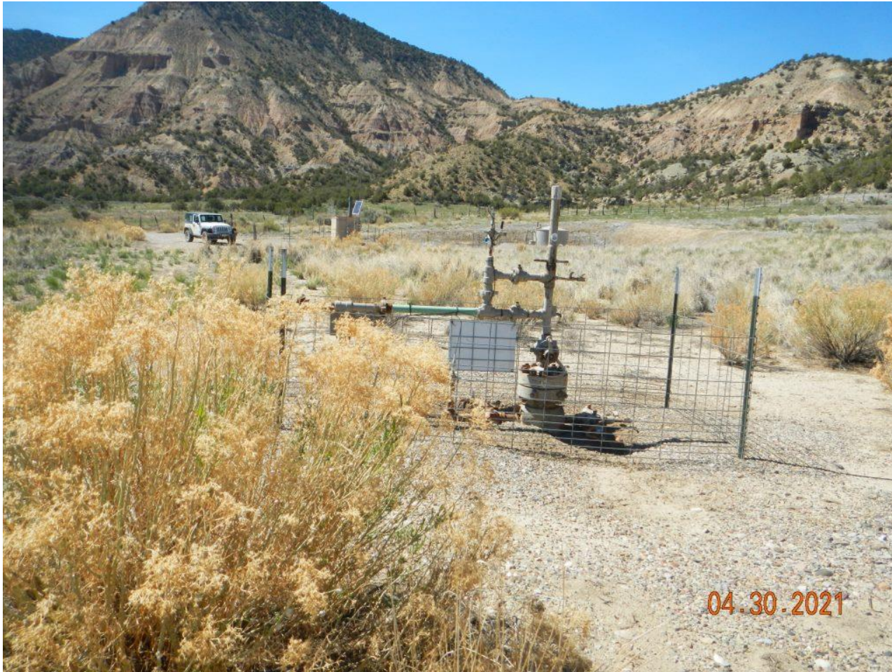
Photo#1: View over Location from Wellhead to entry.
